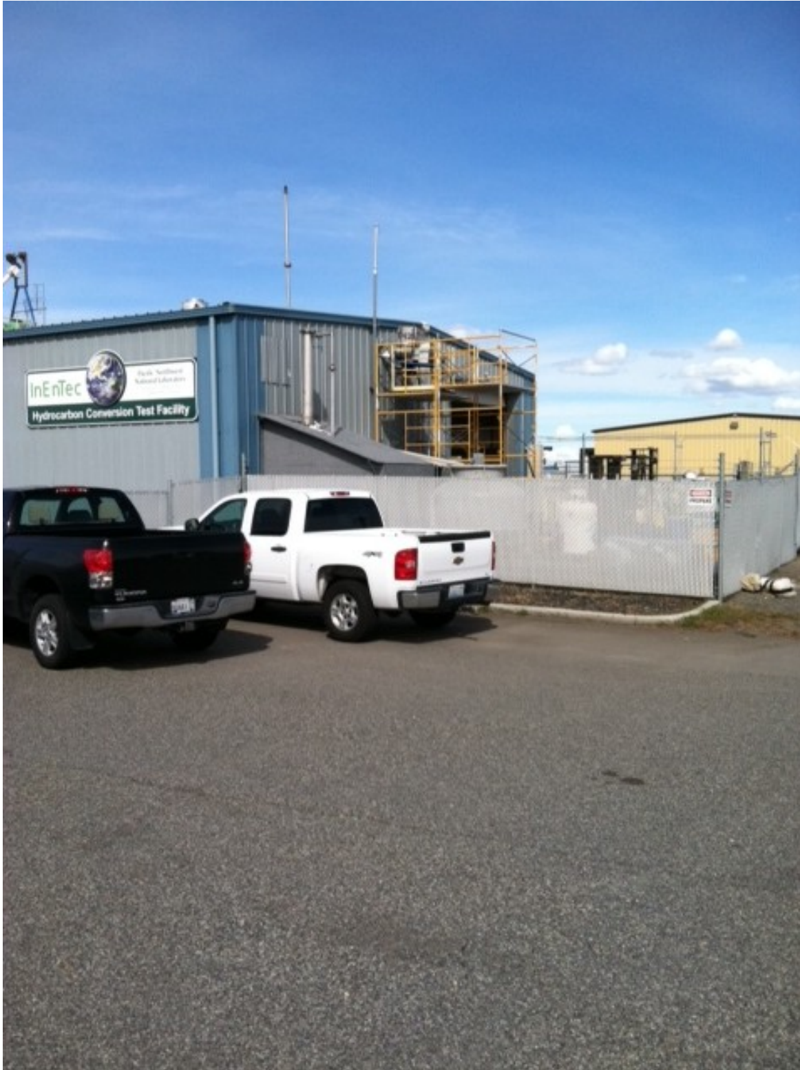
Figure A.2. InEnTec Facility
