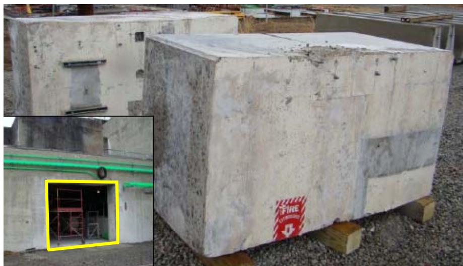
Figure 2-2. Concrete blocks removed from the outer wall of the P Reactor Building with location of wall shown (inset)
