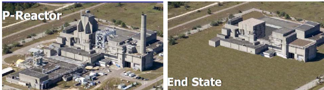
Figure 2-1. The left picture is the P-Reactor Building during its production days and the right picture is a representation of the reactor building after ISD – End State is complete.
