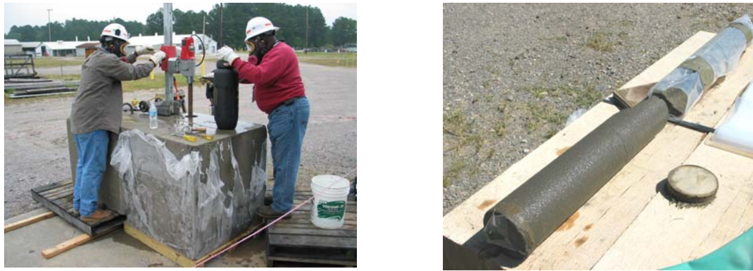
Figure 4-7. Core drilling of the monolith. Samples used for XRD, SEM and strength.
