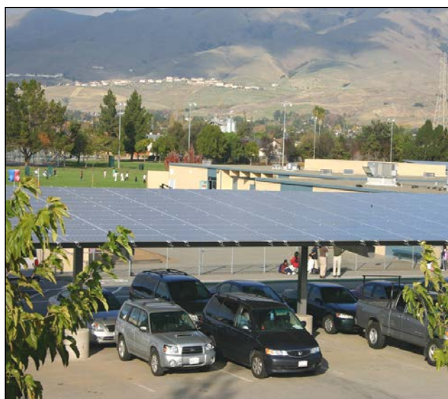
Figure 2. Solar PV array hosted by Milpitas Unified School District. Photo by John Cimino
