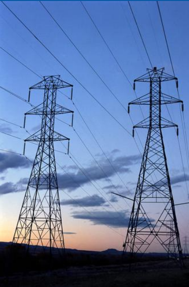
Photo by Warren Gretz, NREL/PIX 00001
