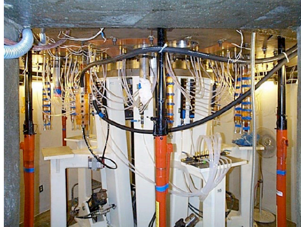
(a) VPI Supply Tubing Under Magnet
