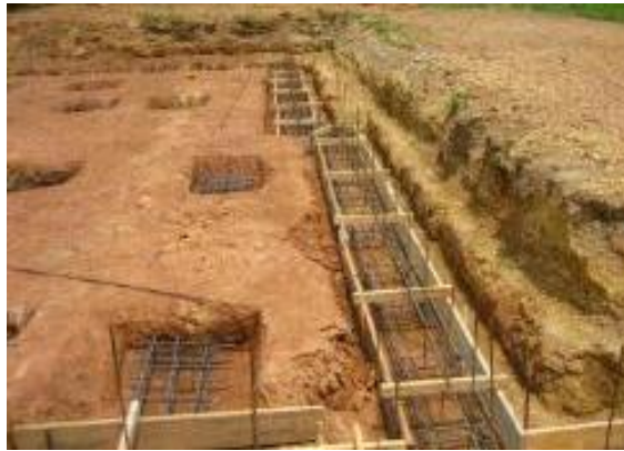
Figure 2. No. 4 rebar used in construction of footer in WC3 and WC4.
