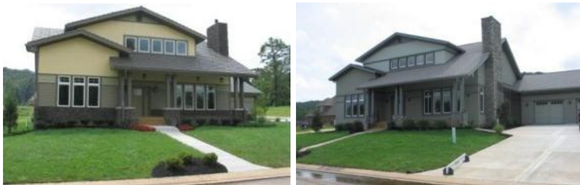
Figure 1. WC3 (left) with vented crawlspace and WC4 (right) with insulated and sealed crawlspace.
