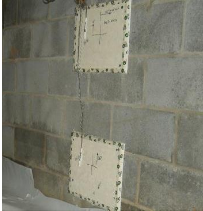
Figure 9. Sensor installation on the WC3 crawlspace masonry wall.
