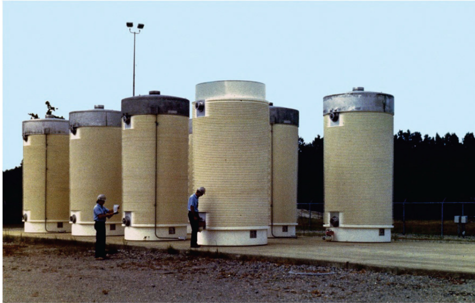
Figure-2: ISFSI with Vertical Spent Fuel Storage/Transfer Casks (Source – U.S. Nuclear Regulatory Commission Library, 2011)
