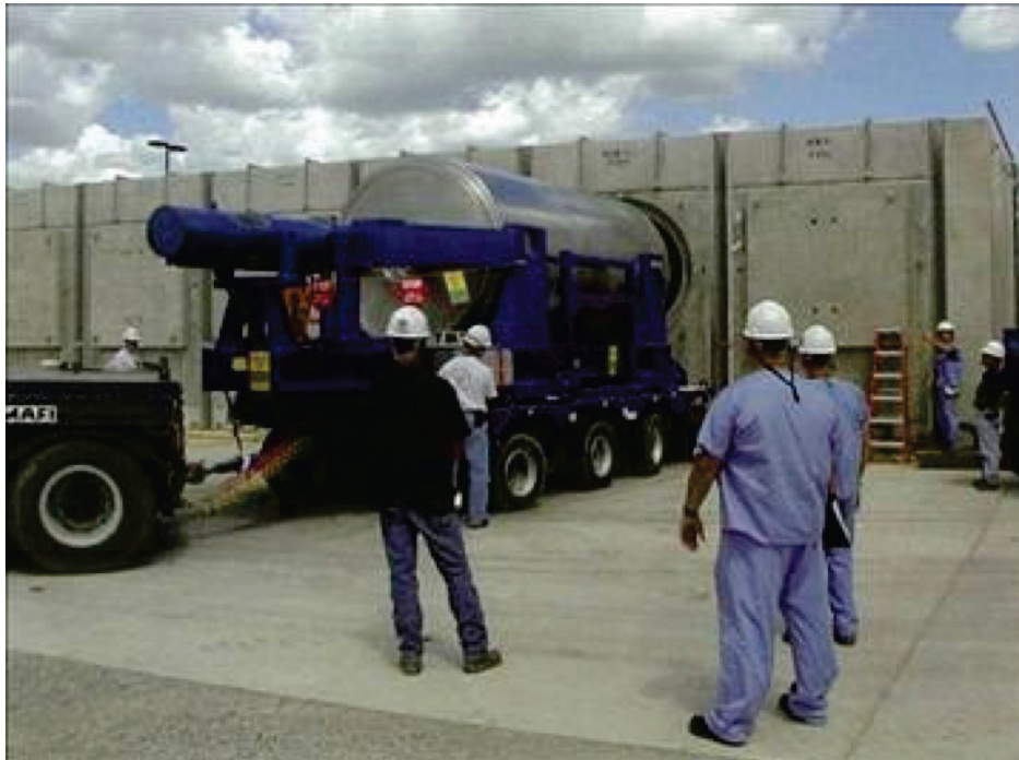
Figure-3: ISFSI with Horizontal Spent Fuel Storage Vault (Source - SFEN Jeune Génération, 2009)
