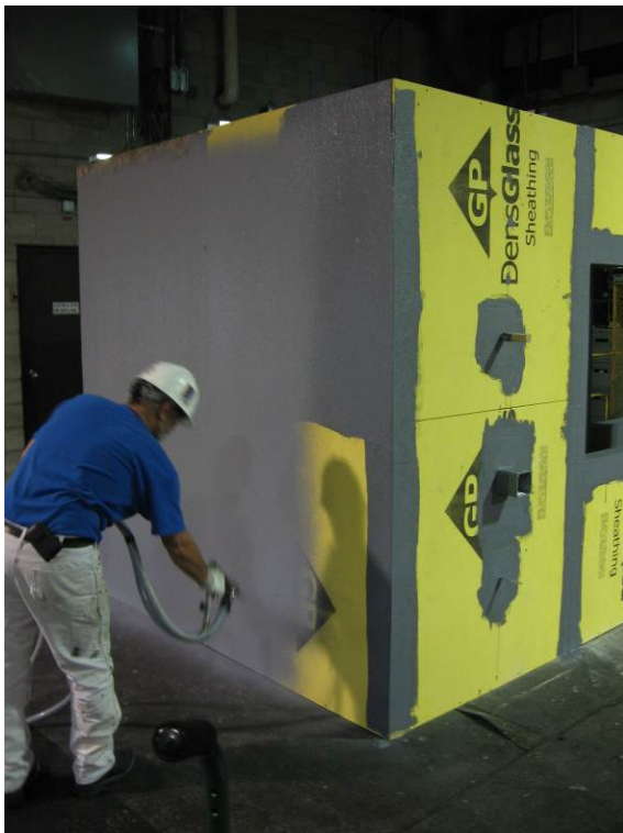
Figure 13. Spray applied liquid applied barrier
