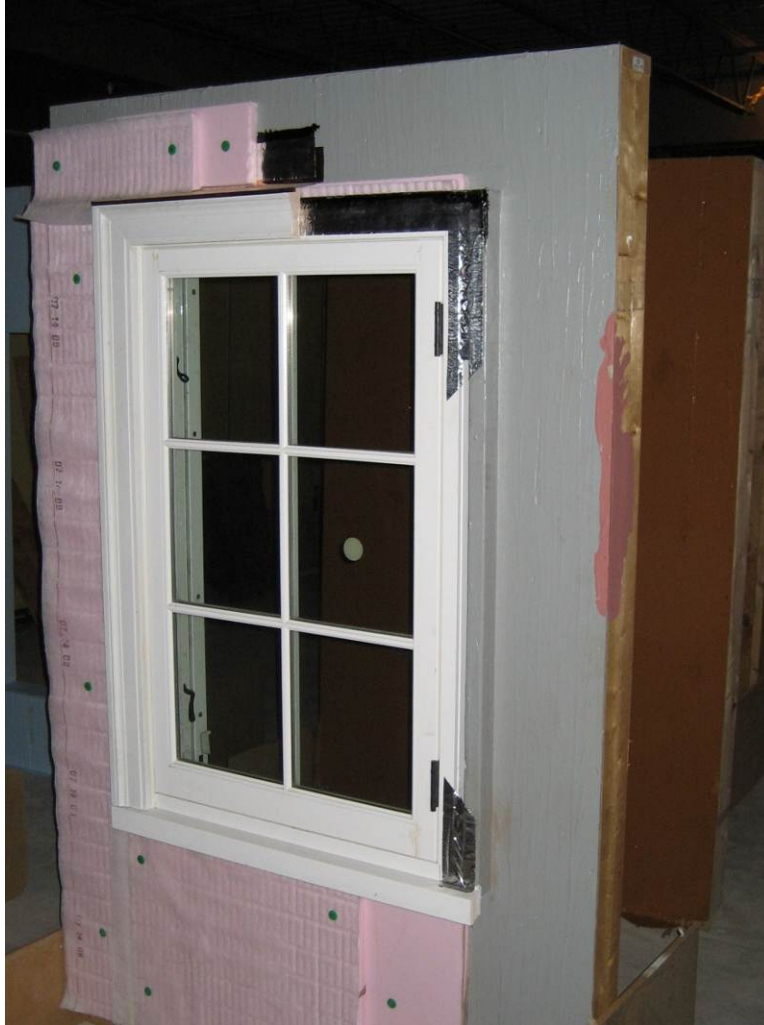
Figure 19. Water management mockup with liquid applied membrane and exterior insulation
