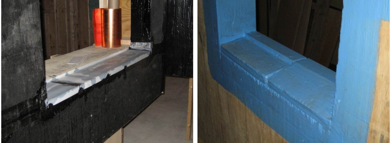
Figure 20. Window sill flashing mockups
