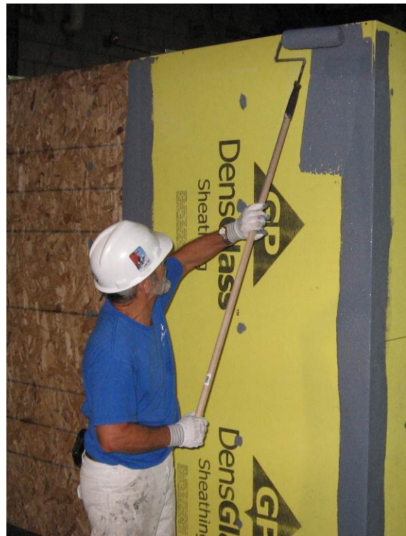
Figure 14. Roller applied liquid applied barrier
