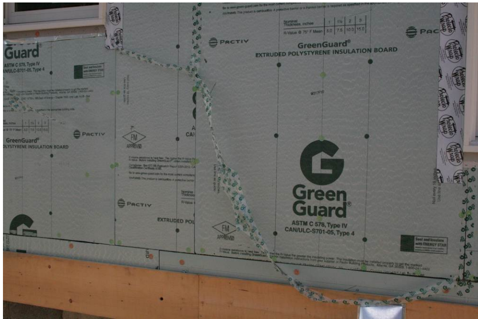
Figure 6. Taped exterior insulation drainage plane
