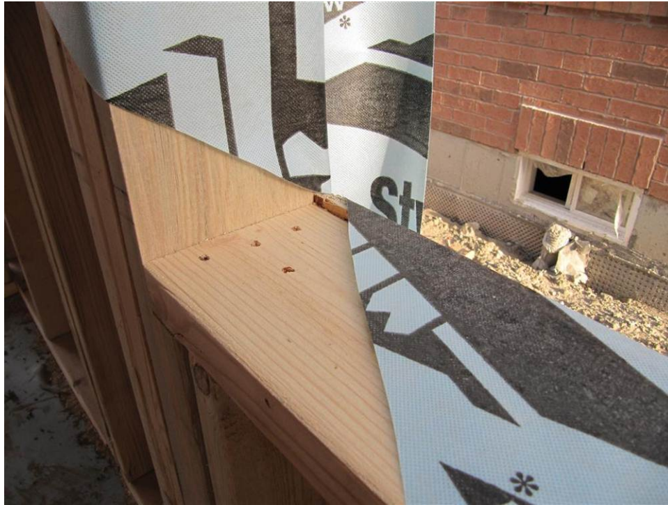
Figure 10. Prepared window opening
