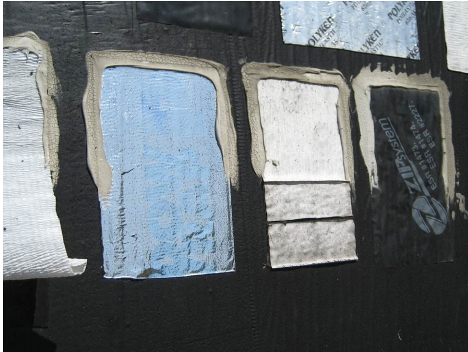
Figure 22. Peel and stick membranes with termination mastic
