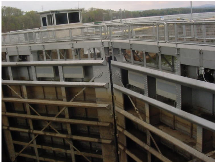
Before and after pictures of the Watts Bar Dam Lock Doors. The Bottom Picture shows the PVT Detectors in the Lock Doors
