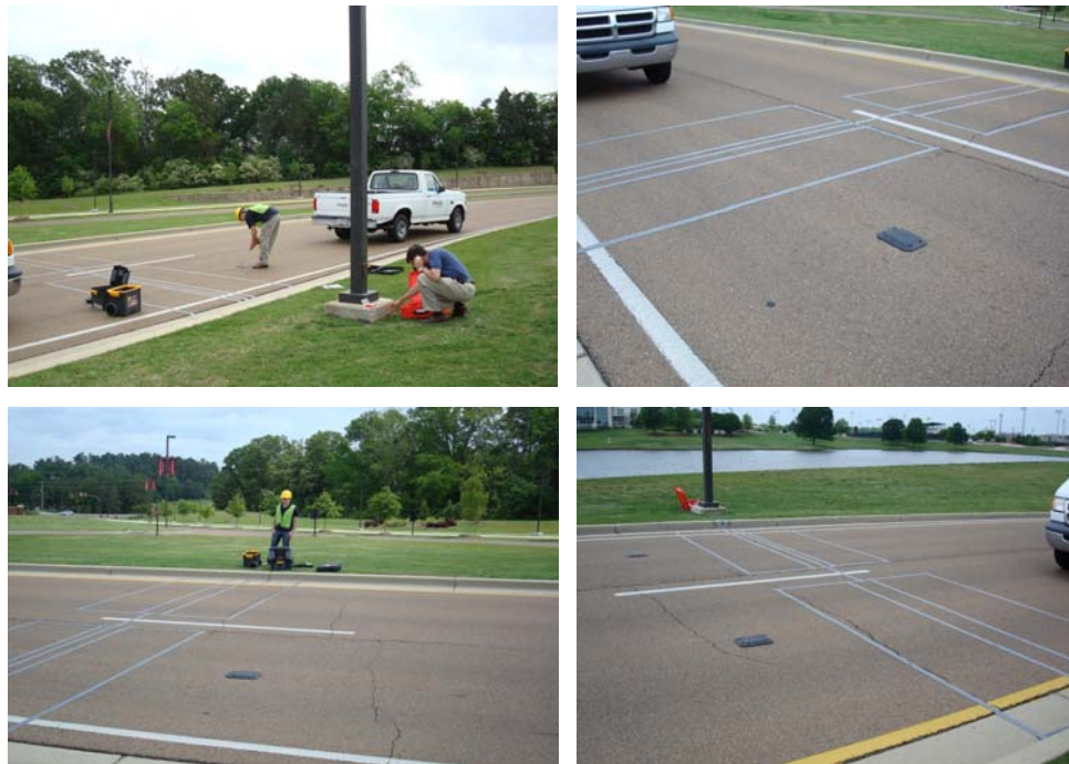
Figure 34 Mississippi FOTs Sensor Deployment (ORNL 1)
