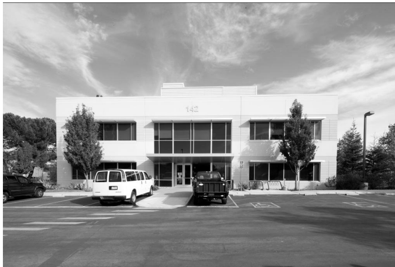
Figure 10. Building 142, office building, 2010
