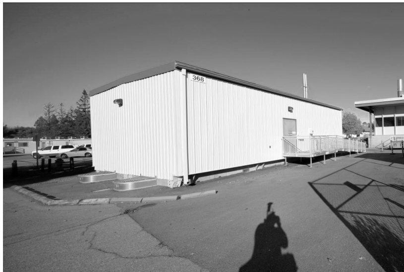
Figure 7. Building 368, BSL-3 laboratory, 2010
