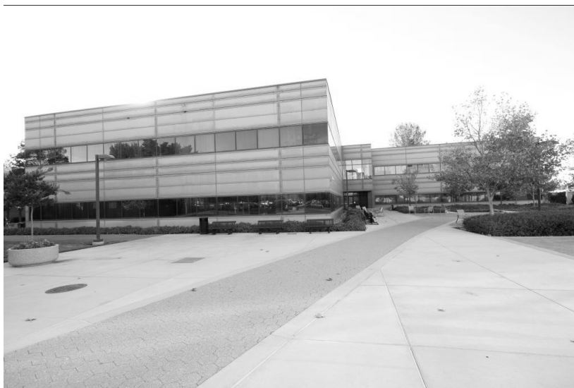
Figure 16. Building 453, Terascale Simulation Facility, north side, 2010
