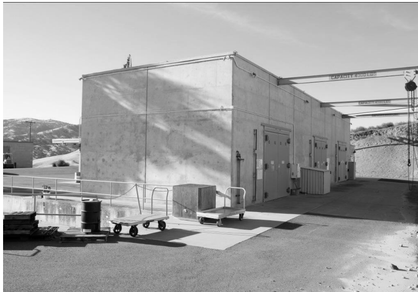
Figure 23. North side of Building 810A, showing assembly cell doors, 2010
