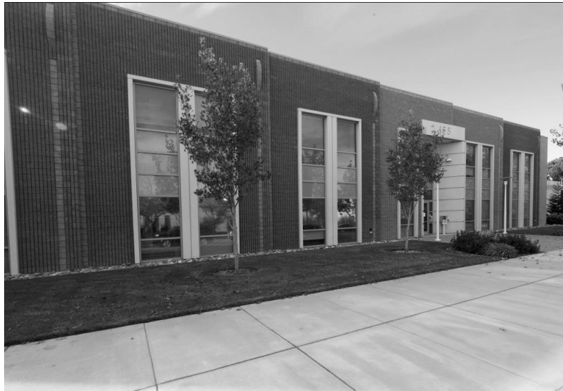
Figure 13. Building 155, ISF offices, 2010
