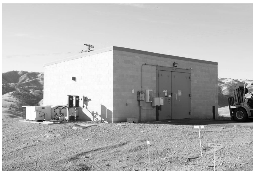
Figure 22. Building 810C, north side, 2010
