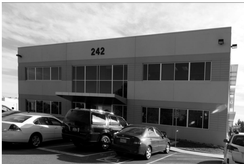
Figure 11. Building 242, office building, 2010
