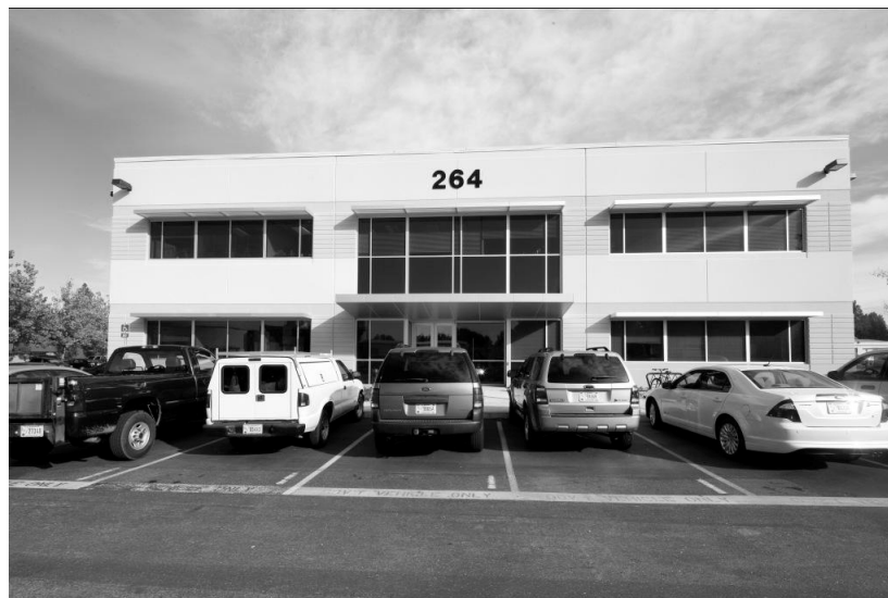
Figure 12. Building 264, office building, 2010
