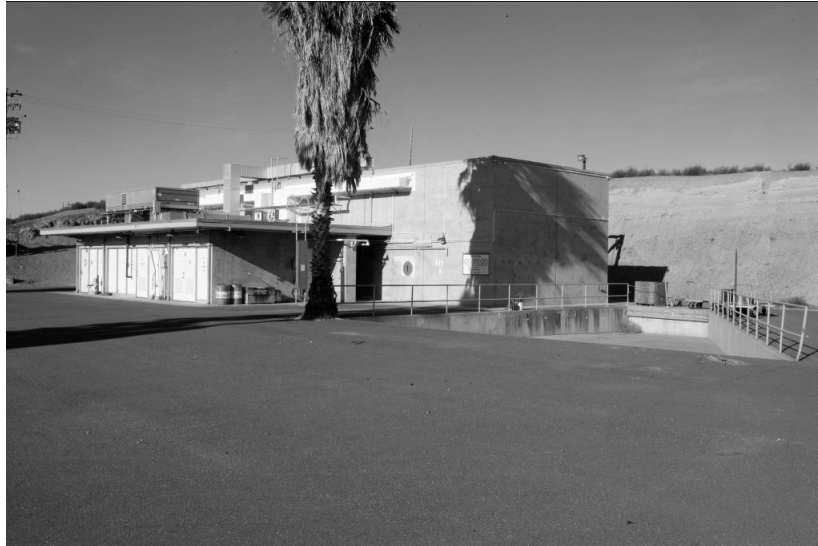
Figure 20. Building 810A, south (front) and east sides, showing both structures, 2010
