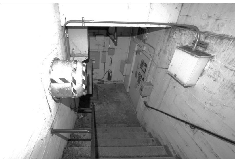
Figure 2. Concrete steps and steel door leading to U-119, 2010
