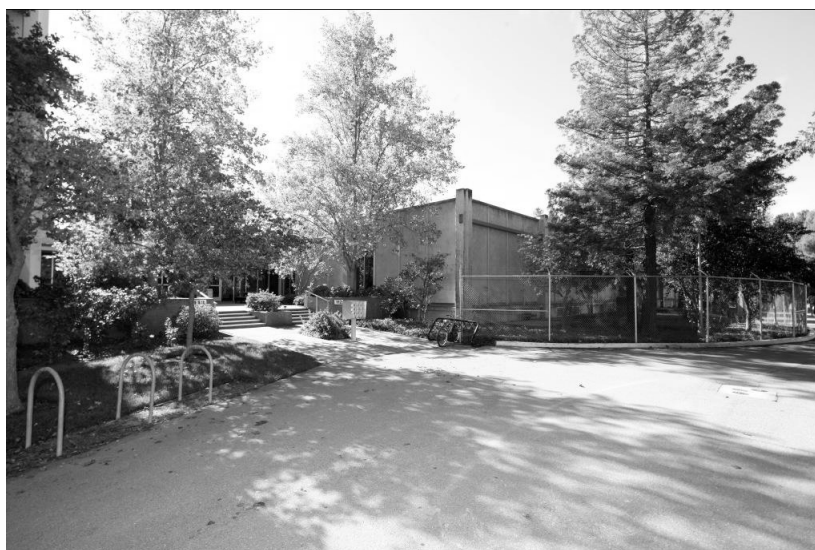
Figure 19. Building 112, computer center, 2010
