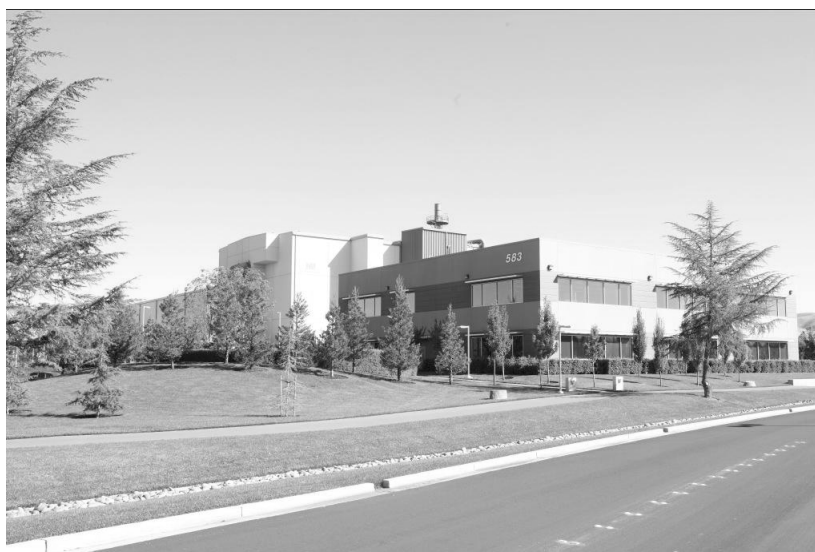
Figure 18. Building 583, NIF offices, 2010
