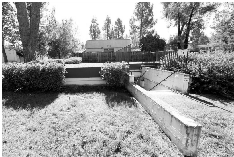
Figure 1. Entrance site to U-119, telecommunications facility, 2010
