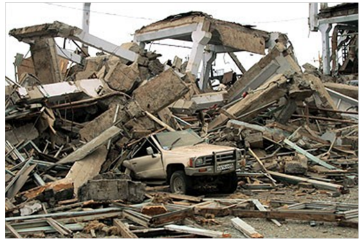
Figure 5. Picture of damage from Nura earthquake. Courtesy www.asiannews.it
