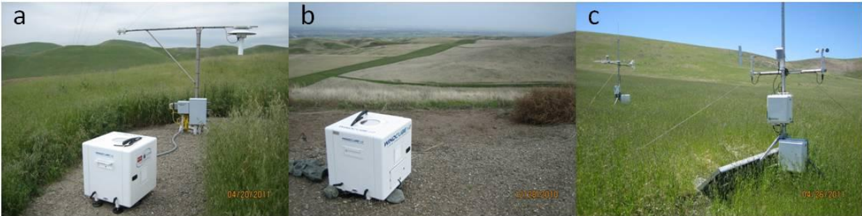
Figure 2: Meteorological instrumentation at Site 300 for the renewable energy program includes (a) LIDAR-96 co-located with the tall meteorological tower at the East Observational Point (EOP), (b) LIDAR-97 near the lightning detector at the EOP, and (c) 3 m tall meteorological and energy flux towers in the valley below. The LIDARs are located on a ridgeline west (and usually upwind) of the flux tower.
