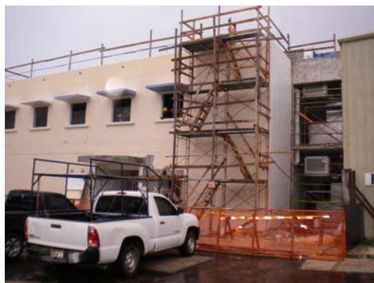
Figure 11. Guam Community College's LEED-registered building under construction
