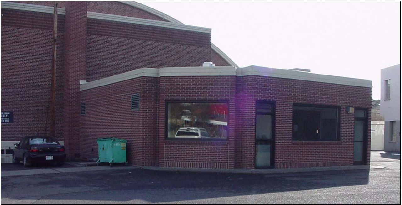
Figure 9. Exterior view of the Geothermal District Heat Center
