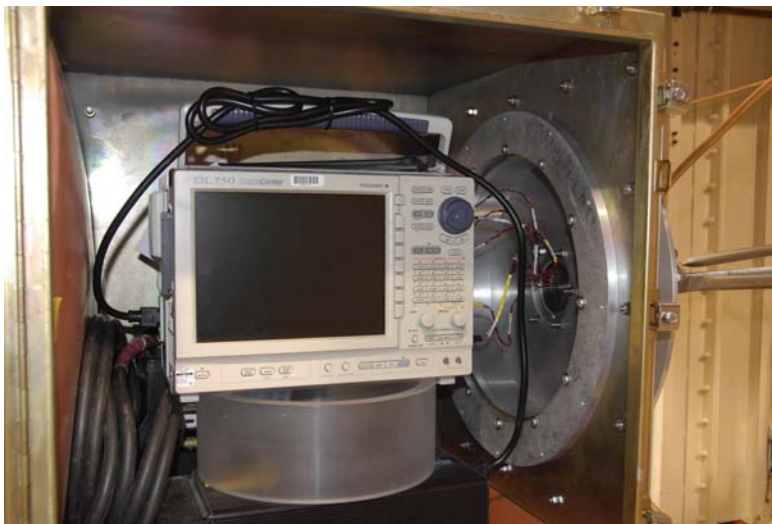
Figure 203. Inside of measurement box showing voltage waveform recording equipment.
