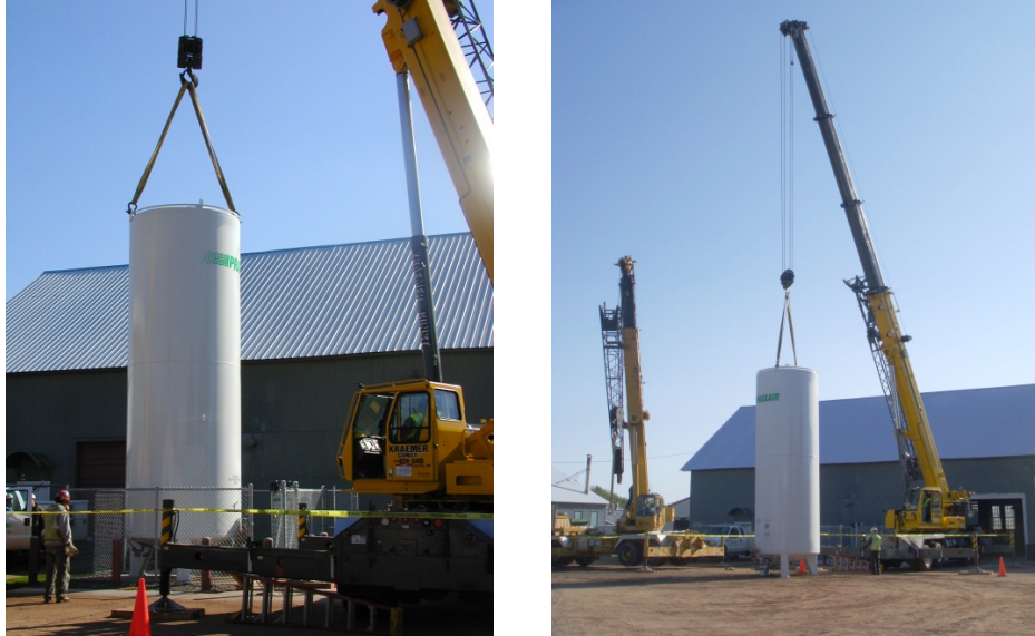
Figure 4-13. Bulk Oxygen Tank Installation
