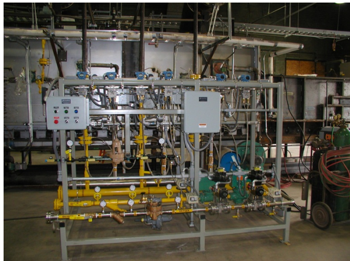
Figure 4-14. Oxygen – Fuel Combustion System valve train
