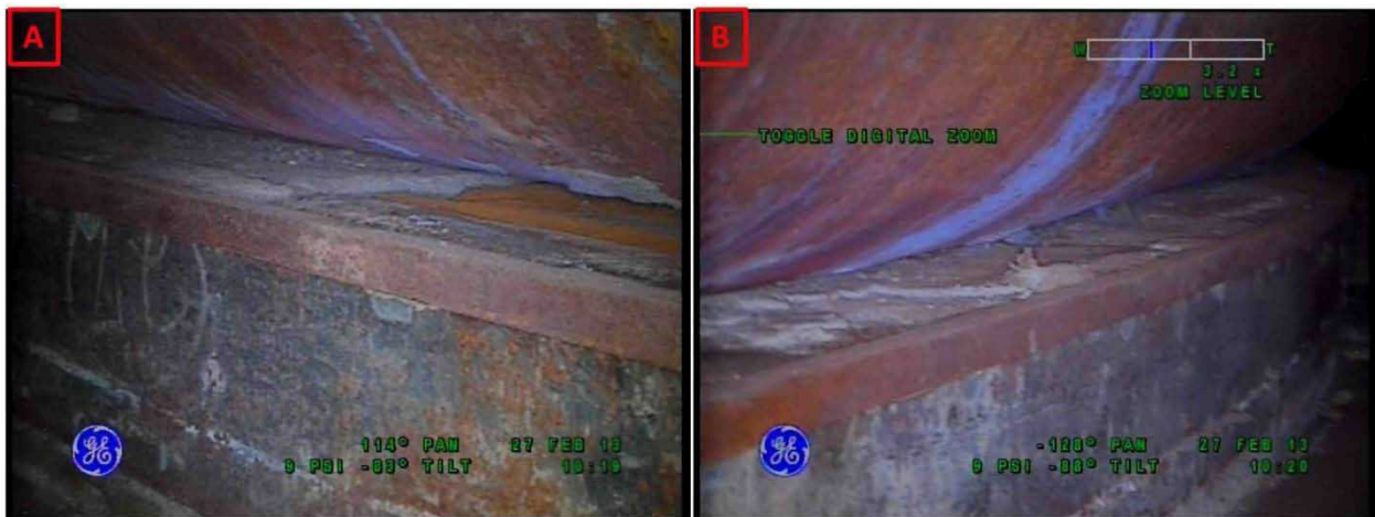
Figure 3-37. Riser 89 General Condition of the Refractory Slots on February 27, 2013
