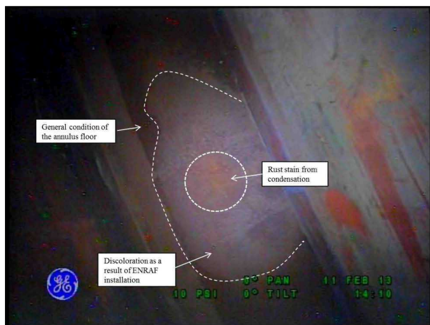
Figure 4-1. Top Down View of the Annulus Floor as seen from Riser 92 on February 11, 2013
