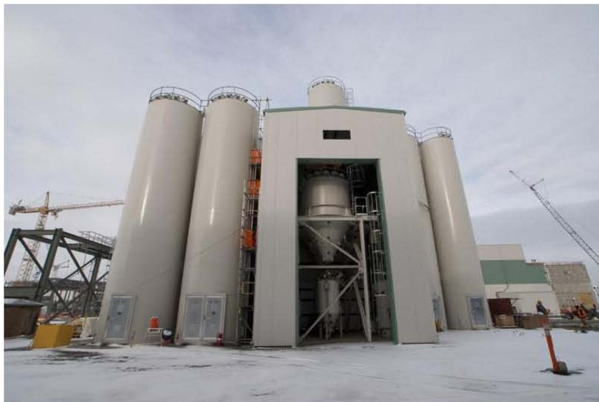
Figure 2-4. Glass Former Facility (WTP December 2009)
