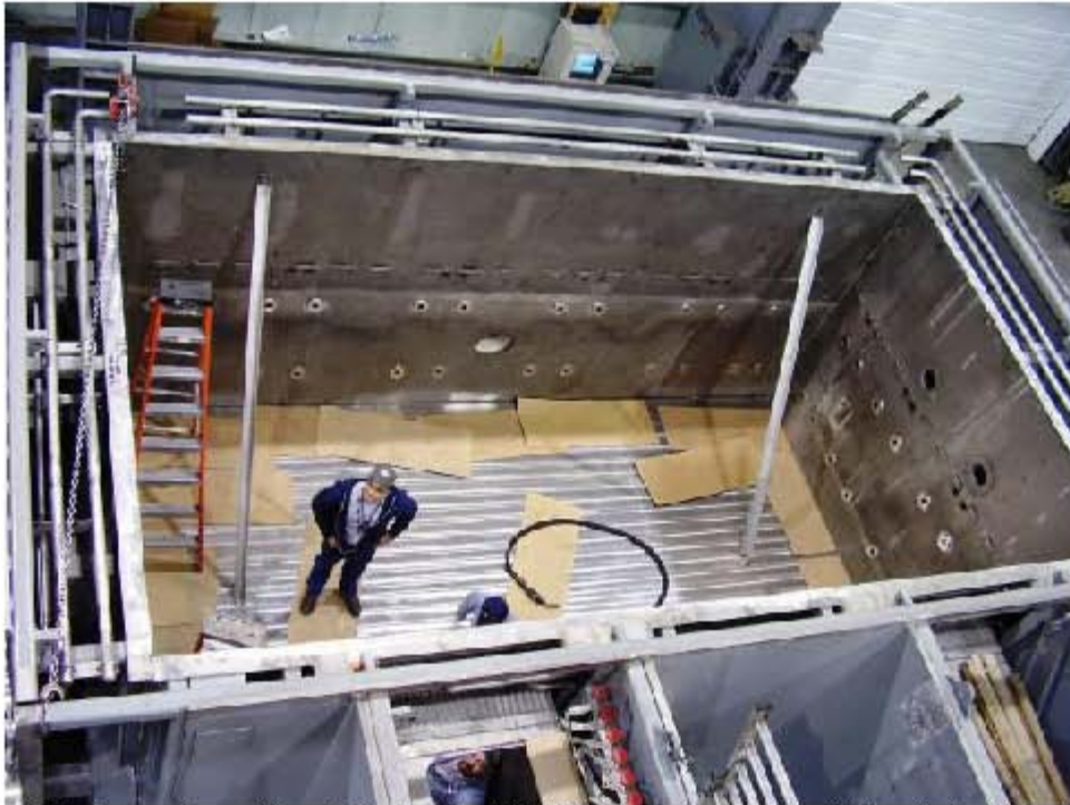
Figure 2-6. LAW Melter under Construction (prior to installation of ceramic lining)
