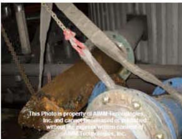
Figure 6-5. Pipeline Blockage or Foulants Handled by the Hydrokinetics System
