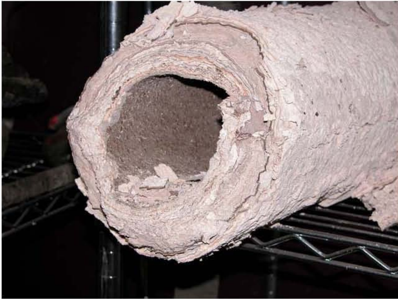
Fig. 12. Calcium carbonate line plug removed using Hydrokinetics™.
