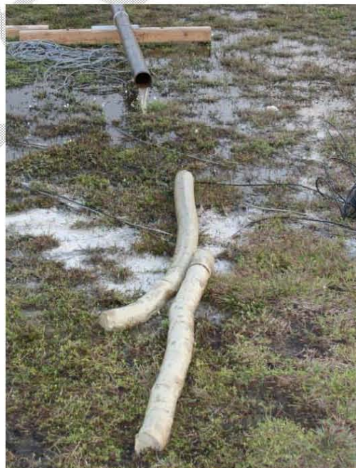
Figure 28. Unplugged 12 ft Bentonite plug (310 ft pipeline).
