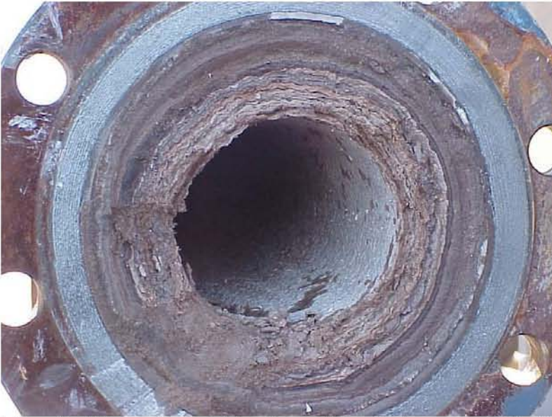
Fig. 10. View of partially plugged line before use of Hydrokinetics™.
