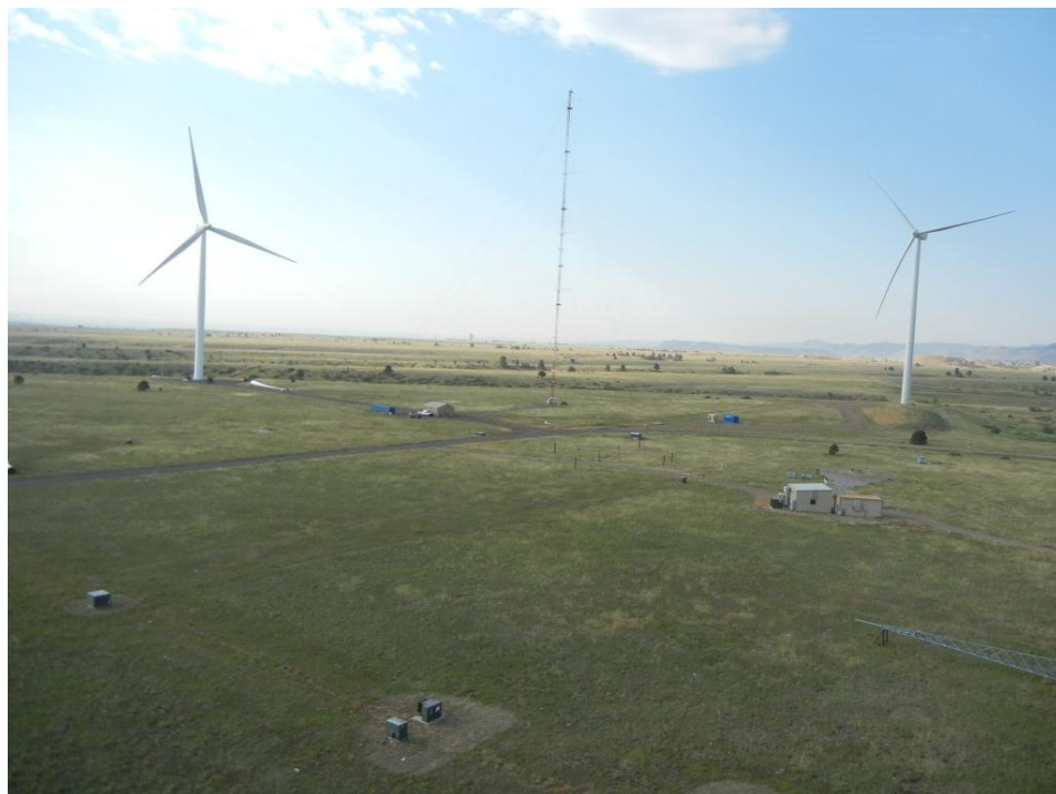
Figure 20. View towards the southeast (Source: NREL 2012)
