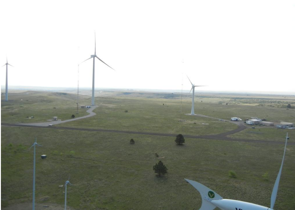
Figure 18. View towards the east/northeast (Source: NREL 2012)
