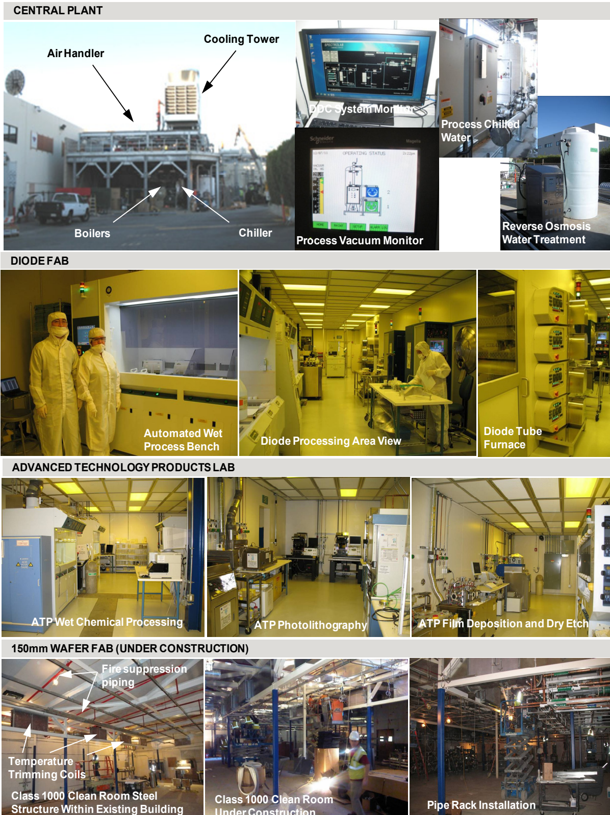
Figure 2-8. Progress toward Completion of the Spectrolab Factory Upgrade
