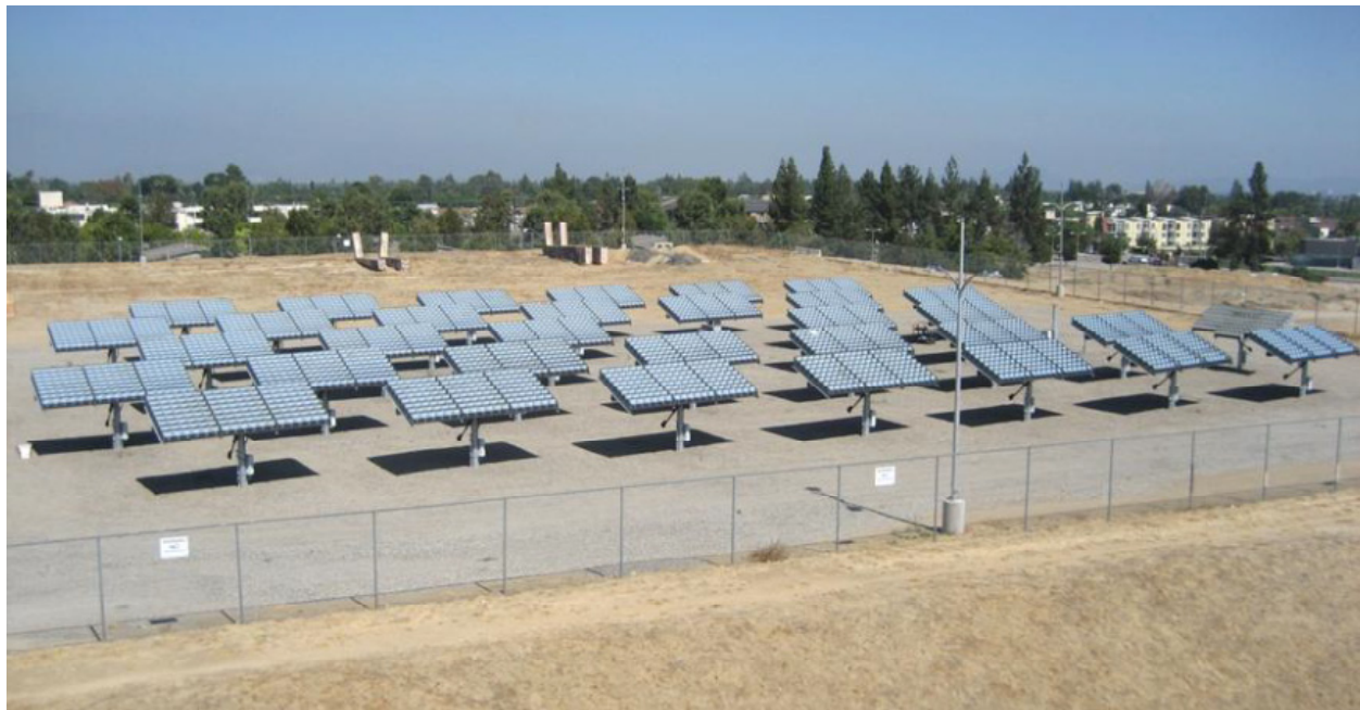
Figure 8-5. CSUN power plant at assembly complete.
