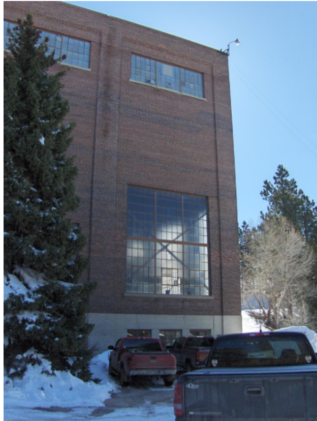
Figure A-17: Photo of Ross Hoist exterior. (HDR)
