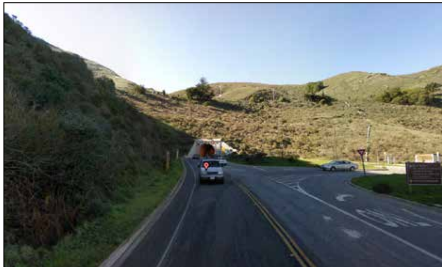
Figure 3.3. View of SE entrance to mountain tunnel (Photo credit: Google)
