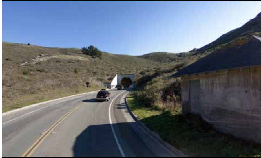
Figure 3.4. View of NW entrance, just past signal (Photo credit: Google)
