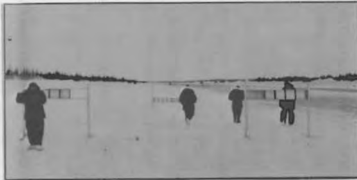
PHOTO SHOWS ERECTION OF VASI SYSTEM AT CLEAR CREEK DURING "BRIMFROST 83"
