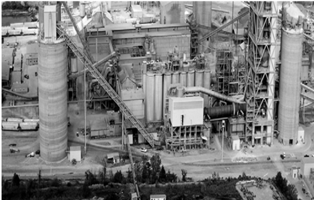
Figure 1-1: Full-Scale Portland Cement Production Facility (Folta 2010)
