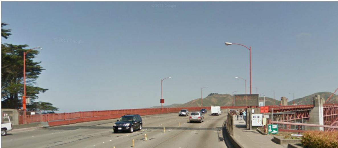
Figure 1.3. First ten cobraheads at south end of bridge (Photo credit: Google)
