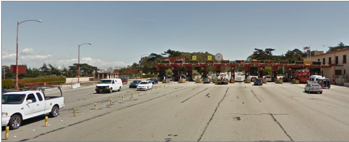
Figure 7.0. Cobraheads just north of the tollbooths (Photo credit: Google)
