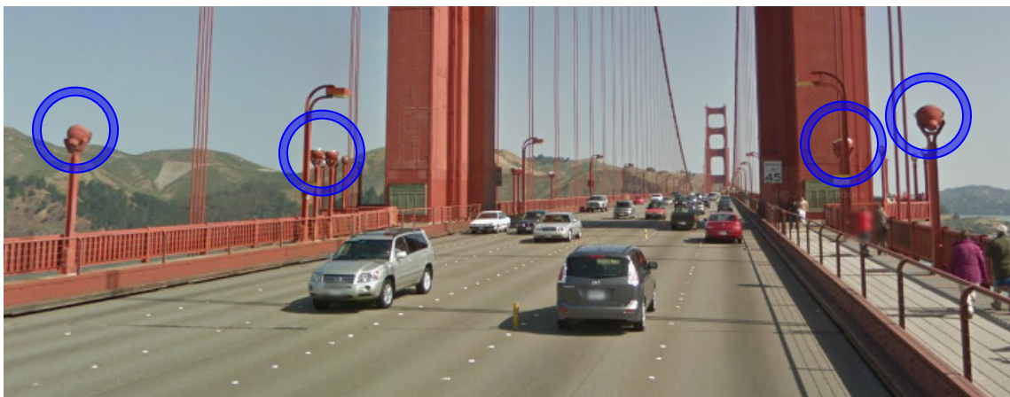
Figure 9.0. One of four possible sets of six floodlights to relamp with CMH (adapted from Google photography)
