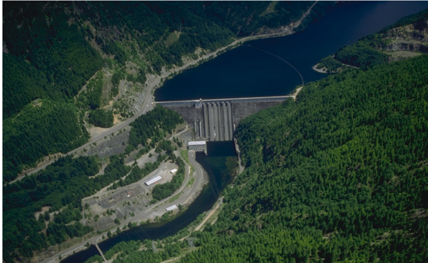
Figure 1.2. Aerial Photograph of Detroit Dam (courtesy of the USACE, http://www.nwd-wc.usace.army.mil/report/det.htm )
