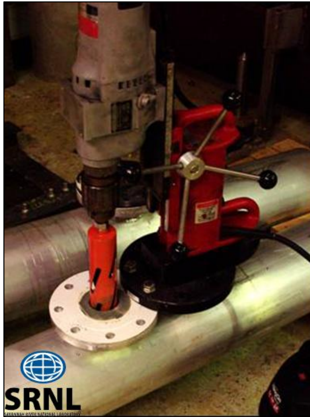
Figure 2-2. Site Port Core Drill Set Up.
