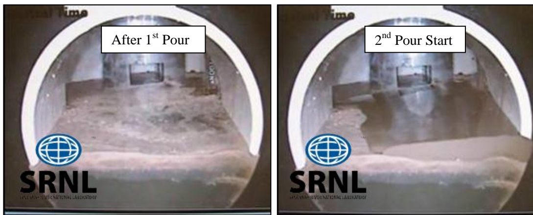
Figure 3-2. Site Port #5 View Between Pours.
