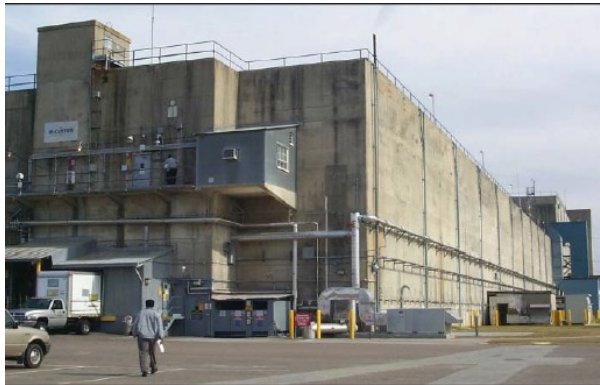
Figure 1. H Canyon Facility at Savannah River Site
