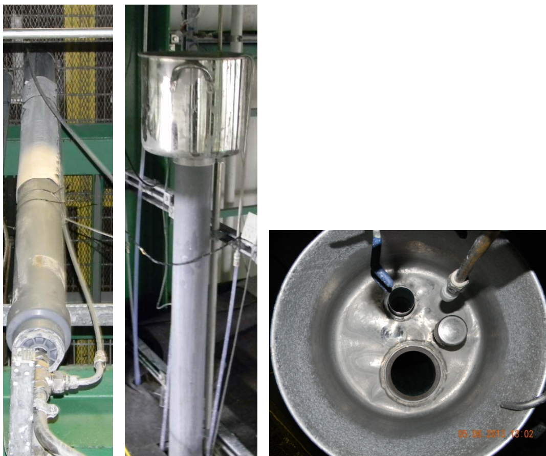
Figure 3-16. De-entrainment Column and Liquid-level Gauge into the Aqueous Head Pot
