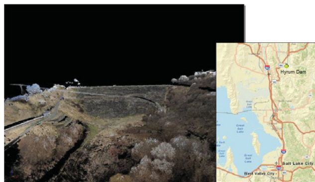
FIGURE 1. 3-D point cloud data and location map of Hyrum dam.
