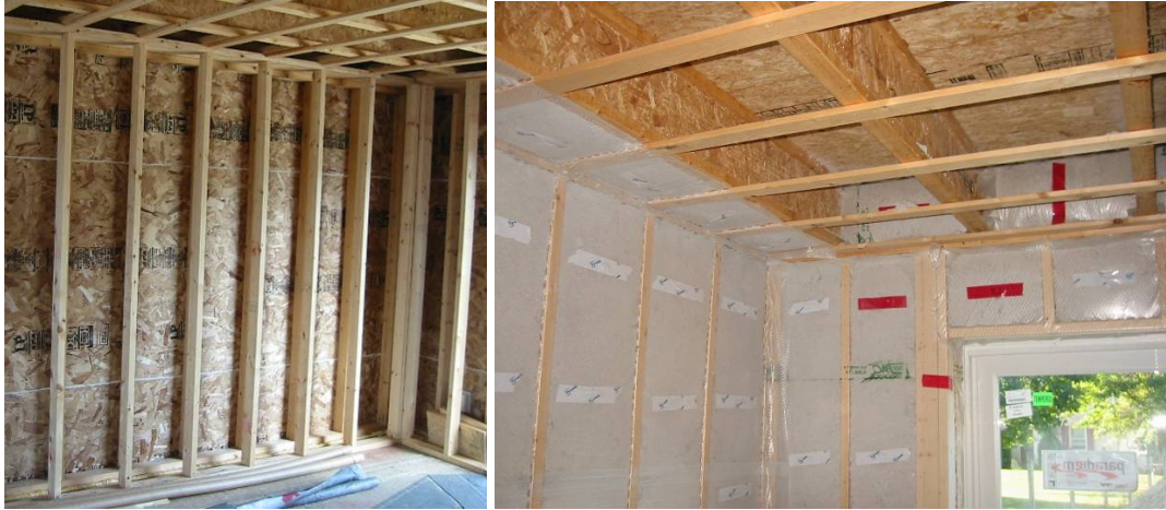
Figure 6. Double walls before and after cellulose insulation.
