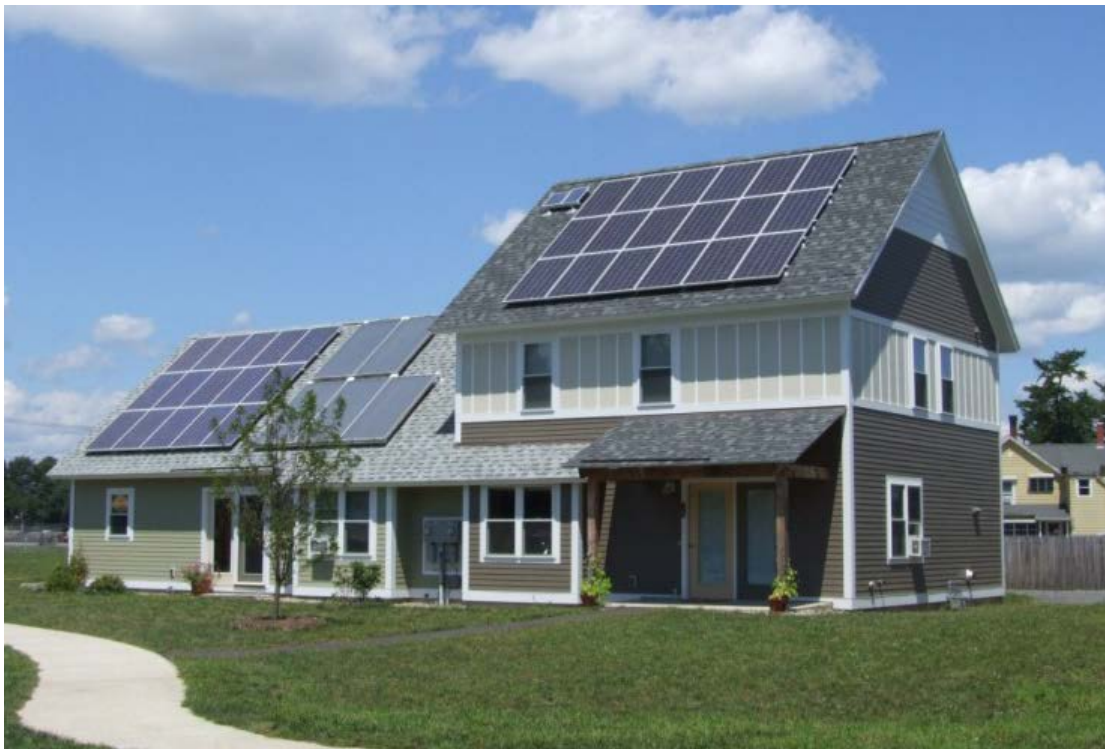
Figure 2. One of the completed WWSV duplexes.
