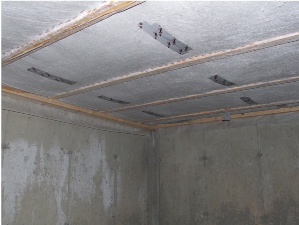
Figure 4. Ceiling of a basement insulated with blown cellulose.
