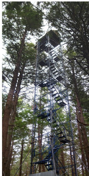
Figure 12. View of the Hemlock tower during the deployment. Photos of the deployment are available at: ftp://boojum.asrc.cestm.albany.edu/pub/HF_WIND_ENERGY/HF_sodar_2011_photos/ .
