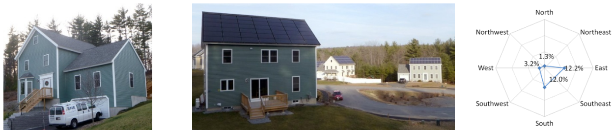
Figure 5. The NZEH in Townsend Left: Northeast view. Middle: South view. The building is part of a low-energy homes development, most of them equipped with PV generators. The room above the garage is unconditioned space. Right: Wall-to-window ratios for different orientations (without garage/extension).
