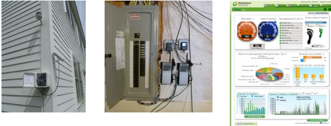
Figure 7. Left: Both homes were equipped with sensors for ambient temperature and RH. Middle: Electric power consumption captured on a circuit level at the breaker box. Right: Electric power consumption visualized on a Web portal.
