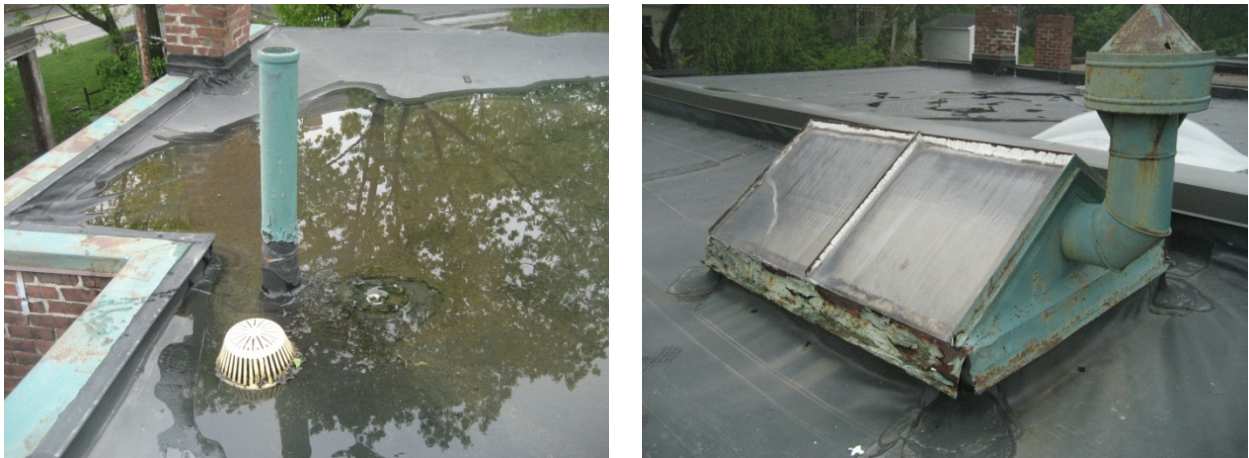
Figure 23. Roof drain (left) and stairway skylight (right)
