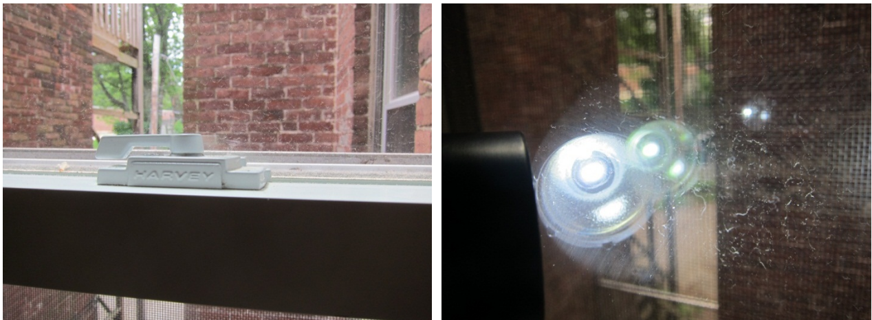
Figure 25. Interior view of the windows and visual inspection of the glass
