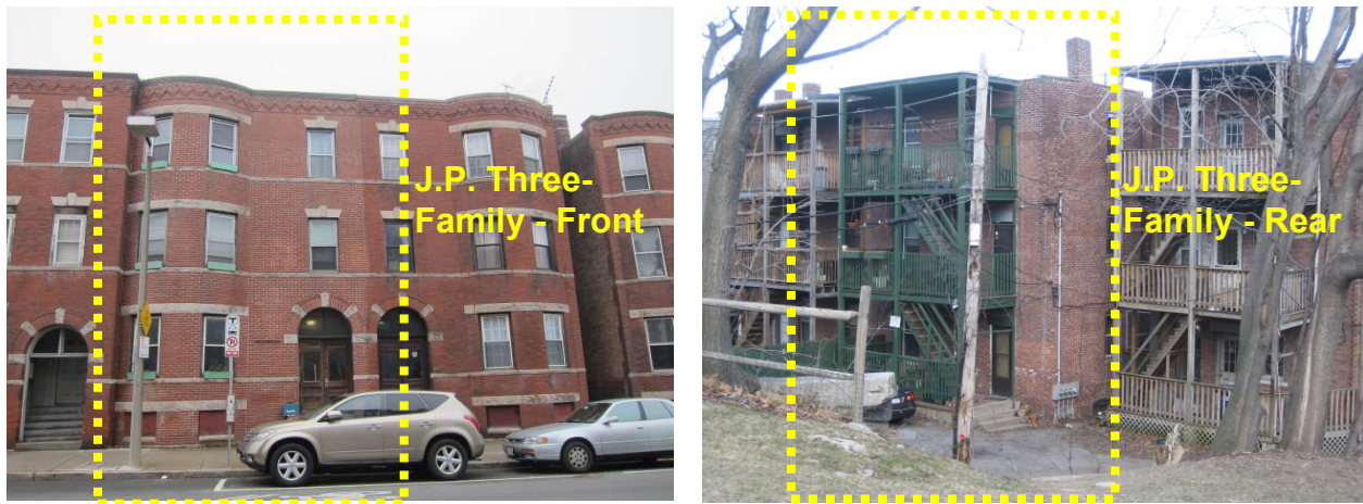
Figure 1. Preretrofit Jamaica Plain Three-Family in Boston, Massachusetts
