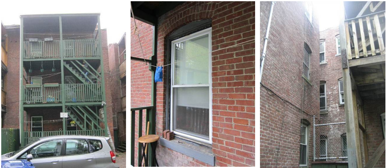
Figure 13. Rear building elevation (left), window detail (center), and light well area (right)
