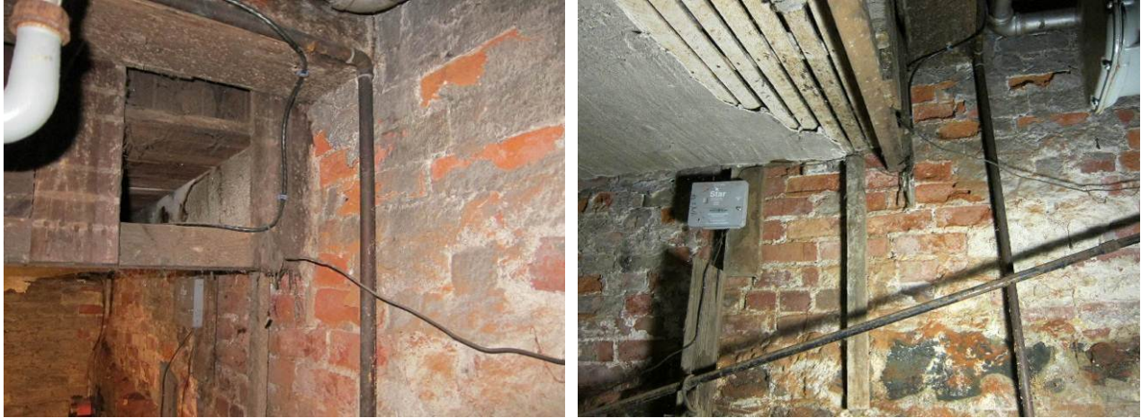
Figure 20. Front entryway wood support structure, with embedment in masonry
