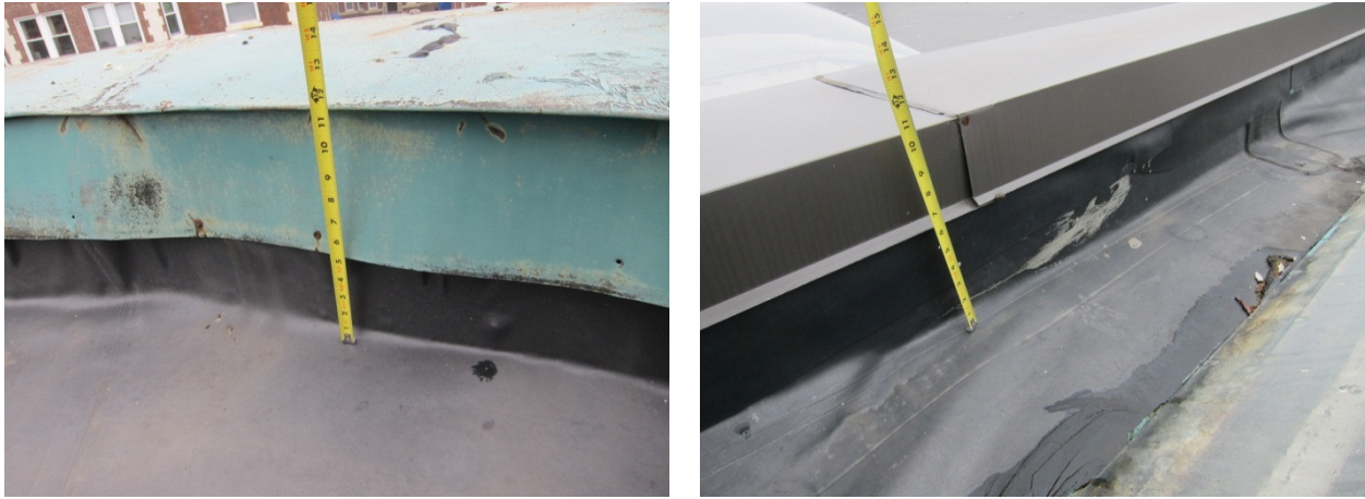
Figure 24. 10–12-in. parapet at front of building (left) and party walls (right)
