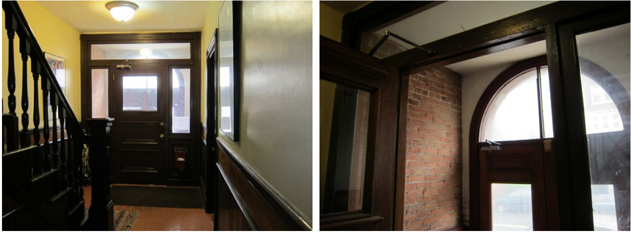
Figure 40. Front door vestibule, showing double doors and glazing
