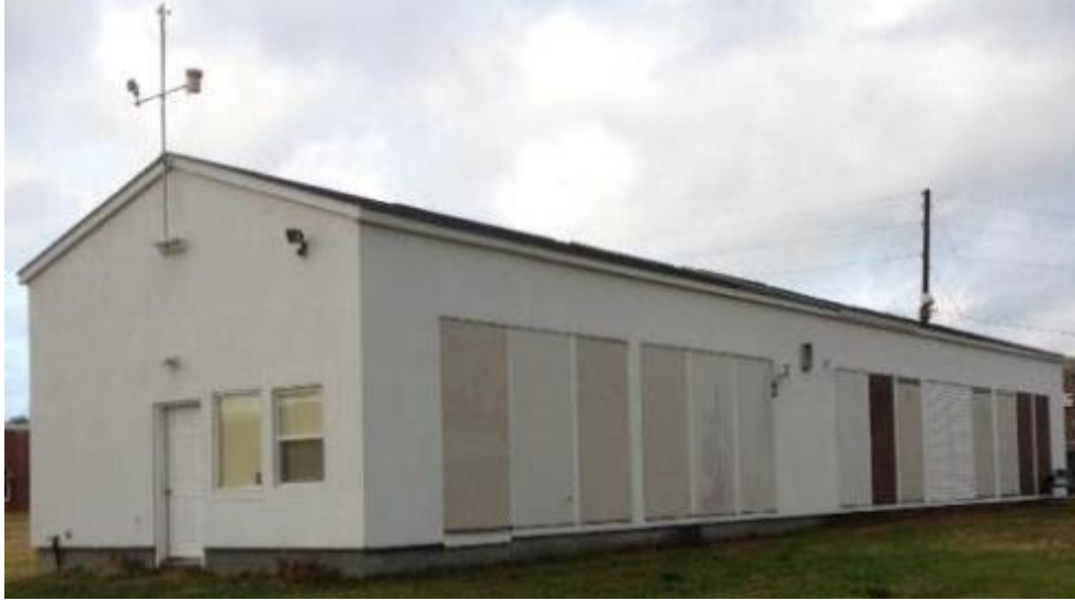
Figure 3. Charleston, SC NET facility.
