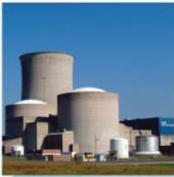
Power uprates and plant life extension
