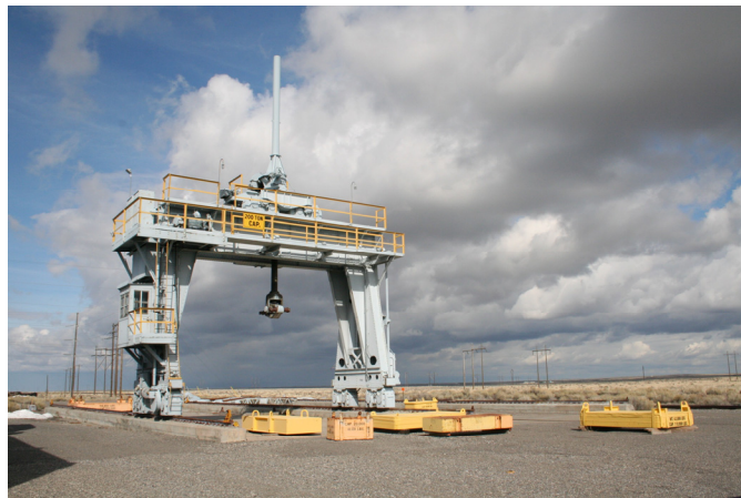
Figure 11. 1943 gantry crane used to offload guns used by the Pacific Naval Fleet.
