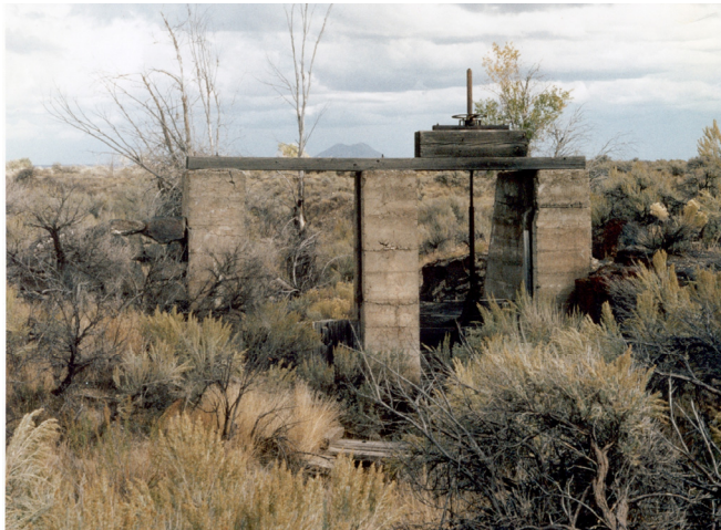
Figure 5. Concrete diversion on the dry Big Lost River, built ca 1910.
