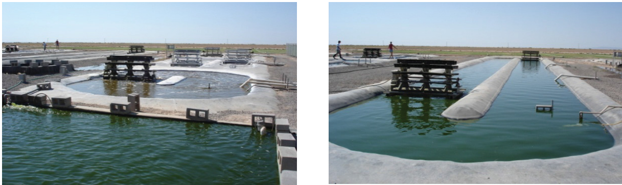
Figure 7. Example of pond construction (<10-acre ponds) (Pecos, TX).
