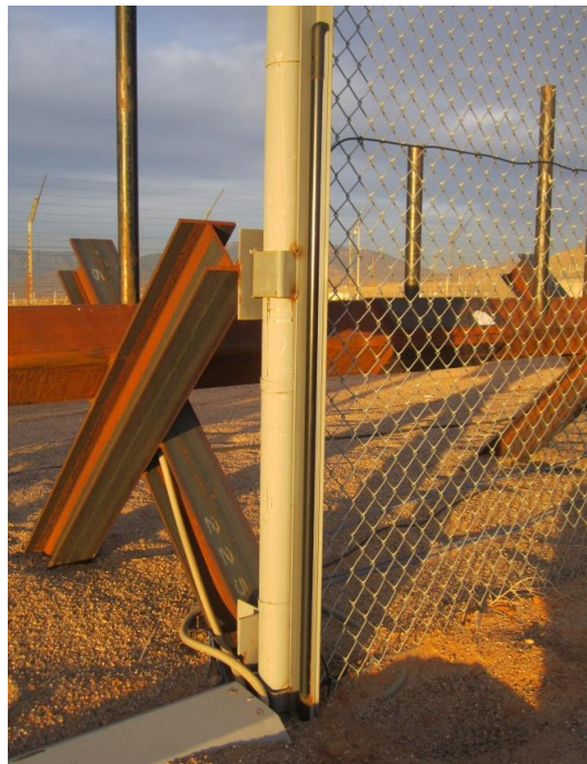
Figure 5: Photon Installation Configuration
