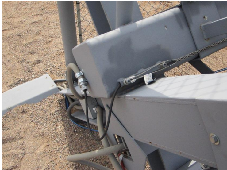
Figure 20: LightLOC Conveyance through Maintenance Access Portal
