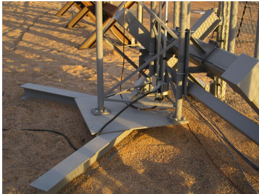
Figure 15: Tower Integration with the Barrier
