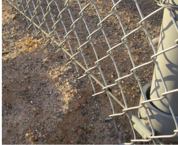
Figure 10: Bottom Tension Wire Installation
