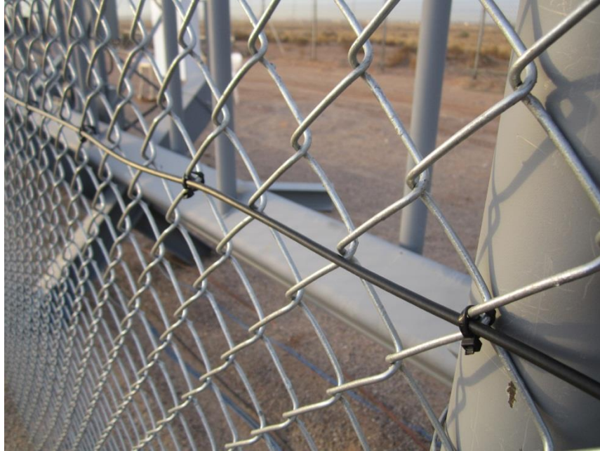
Figure 8: MicroPoint Installation on Fence
