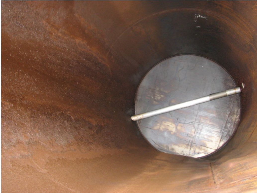
Figure 4. MFC Biodiesel Underground Storage Tank after Cleaning
