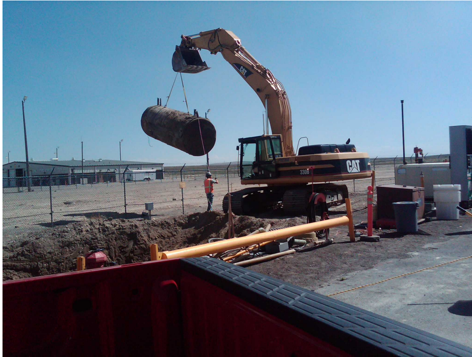
Figure 1. MFC Biodiesel Underground Storage Tank Removal.
