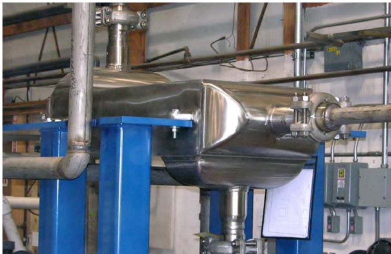
Figure 2-8. S-CO 2 high-temperature PCHE recuperator.
