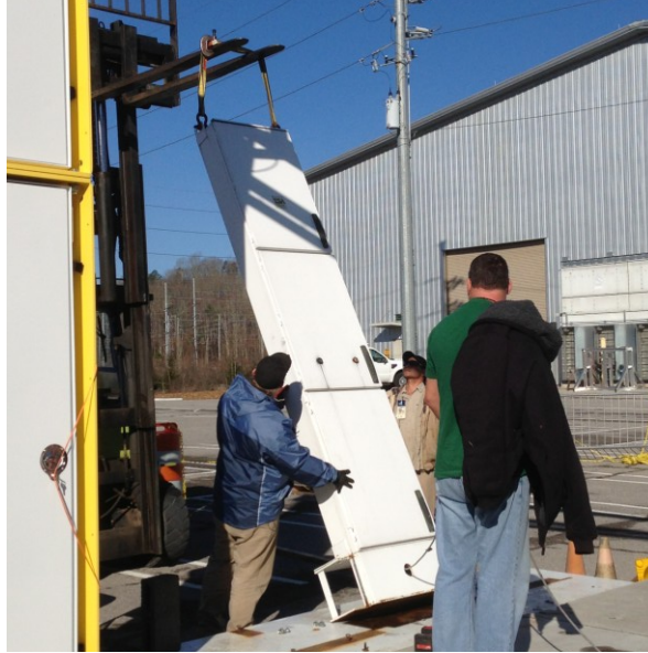
Figure 5. Rigging crew lowering the RPM pillar for collimator installation.
