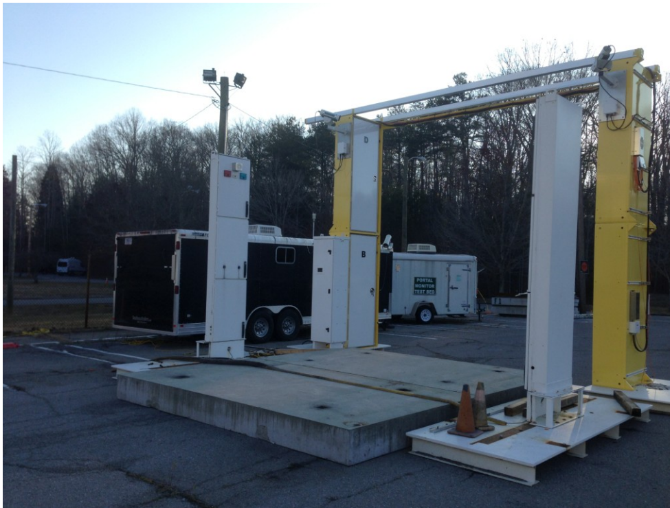
Figure 2. Concrete slab between RPM pillars.
