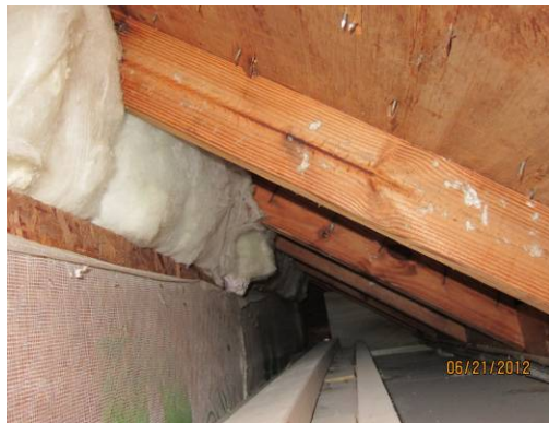
Figure 21. The old soffit is a major leakage pathway as a result of an access opening being cut out between the two attic spaces to allow for the dehumidifier ductwork to run to the existing portion of the home.
