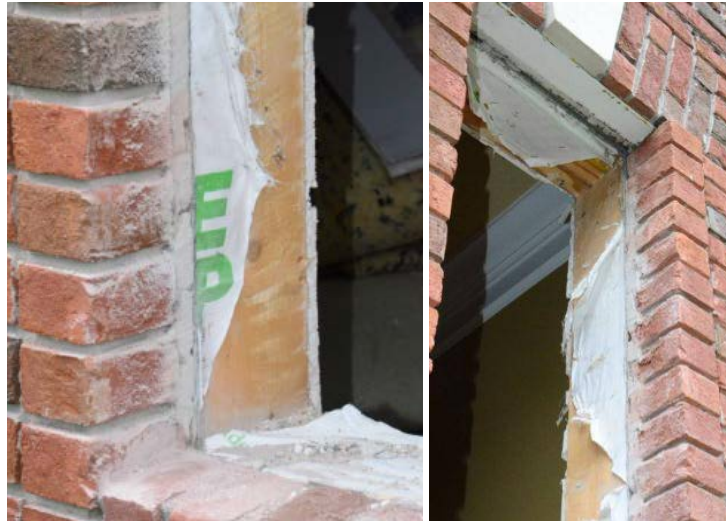
Figure 11. Rough opening after window removal [Images courtesy of BARA]
