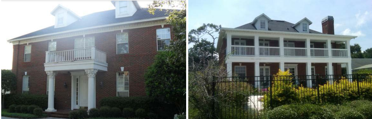
Figure 1. Front (west) and rear (east) elevations, pre-retrofit
