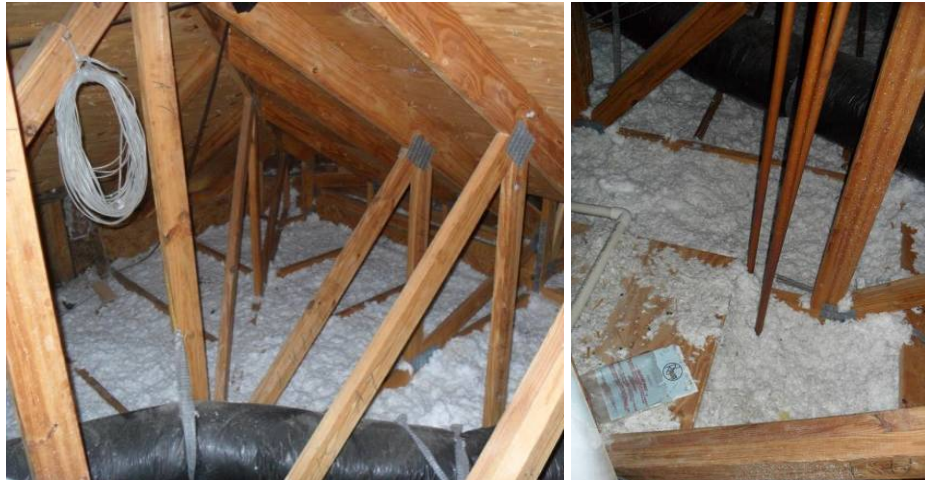
Figure 9. Attic floor insulation, pre-retrofit
