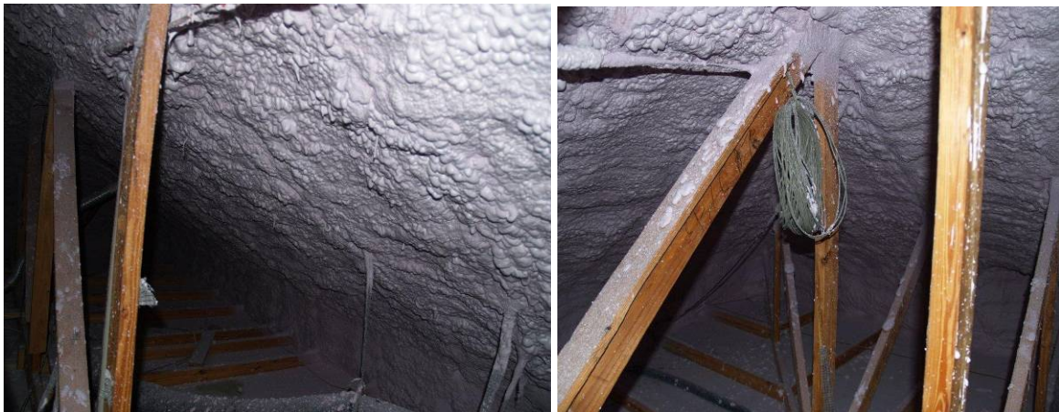
Figure 10. Attic roof deck insulation, post-retrofit [Images courtesy of BARA]
