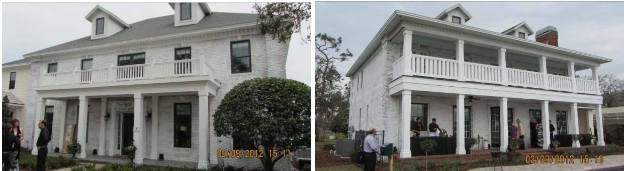
Figure 2. Front (west) and rear (east) elevations, post-retrofit
