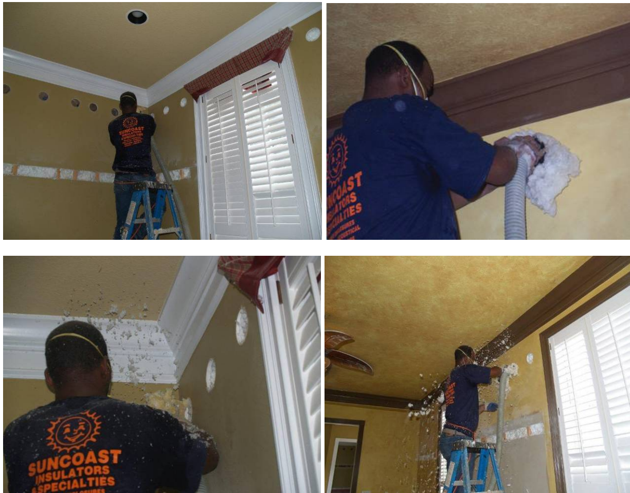
Figure 8. Process of insulating the walls [Images courtesy of BARA]
