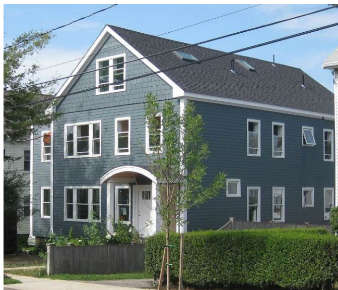
Figure 13. The post-retrofit Belmont Two Family
