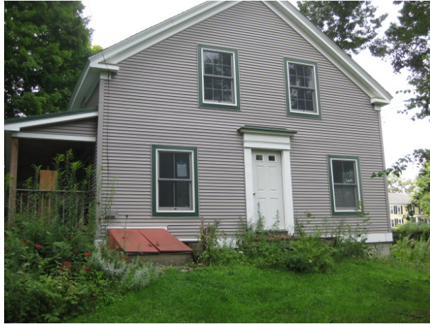
Figure 9. Pre-retrofit Belchertown Cape
