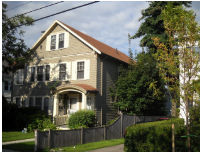
Figure 12. The pre-retrofit Belmont Two Family
