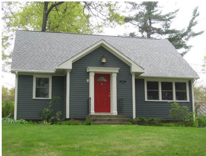
Figure 17. Post-retrofit Millbury Cape
