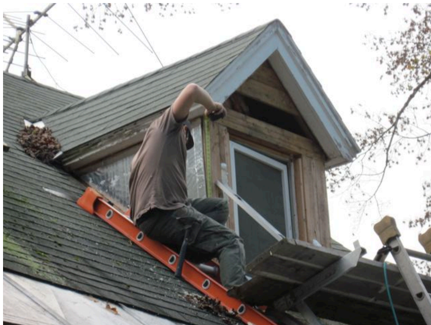
Figure 20. Dormers wrapped in foam (Courtesy of Mindel and Morse Builders)
