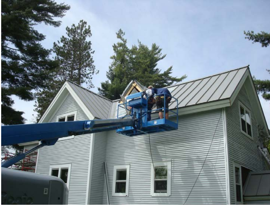
Figure 29. SIP retrofit panel installation with double fascia
