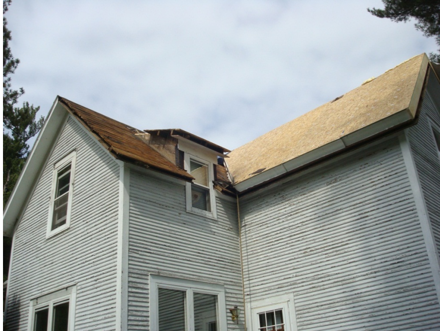
Figure 27. SIP retrofit panel installation
