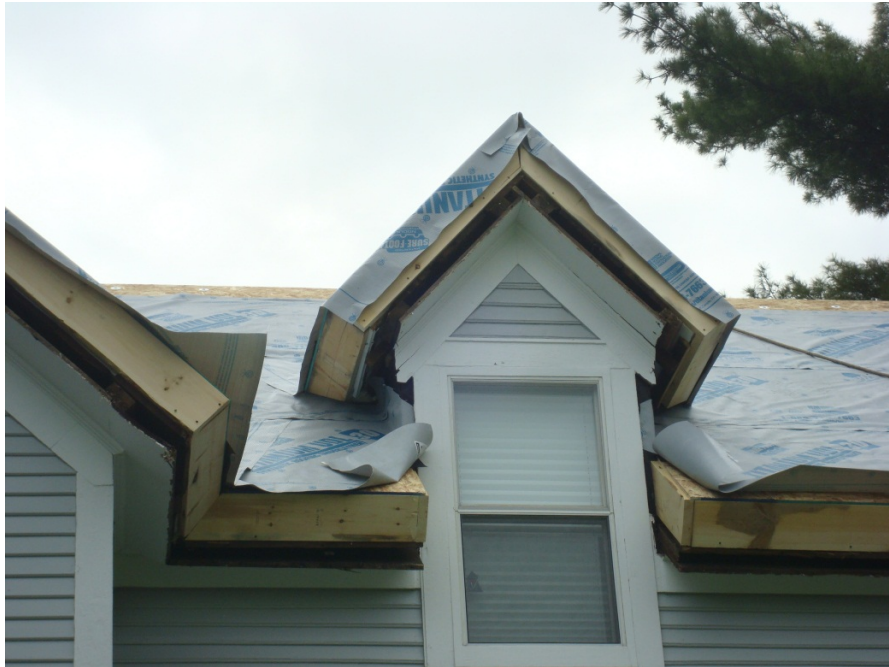
Figure 28. SIP retrofit panel installation over dormer
