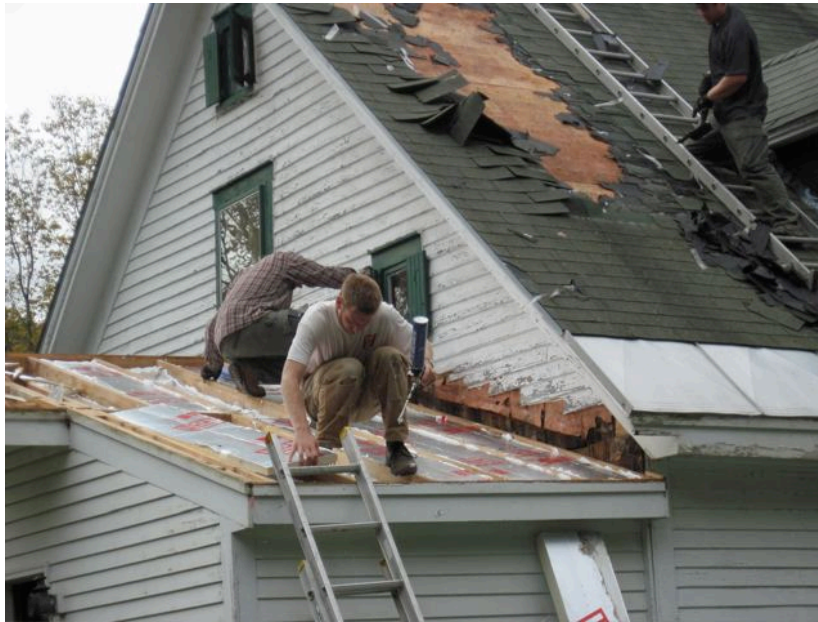
Figure 19. Foil-faced foam between rafter framing (Courtesy of Mindel and Morse Builders)
