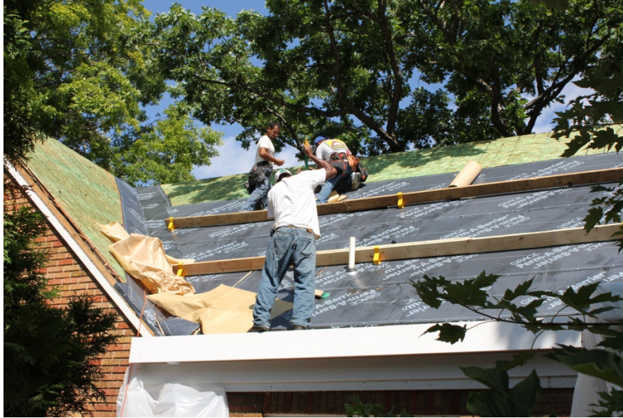
Figure 24. Installing the air/vapor barrier over existing roof decking (Courtesy of Cocoon)
