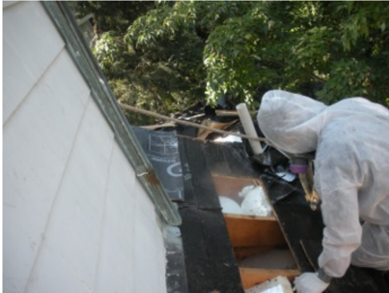
Figure 18. Exposing rafter cavities to prepare for spray foam insulation
