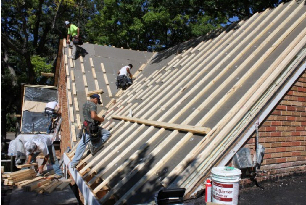
Figure 26. Ventilation of ETMMS
