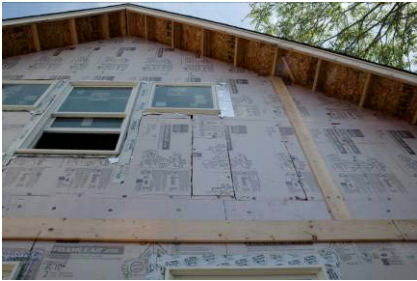
Areas in the field of the wall that require tape sealing
