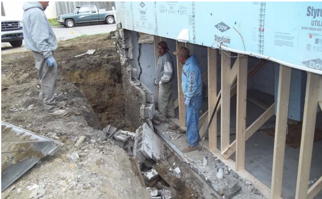
Figure 5: Repair work on Cedar 2 foundation
