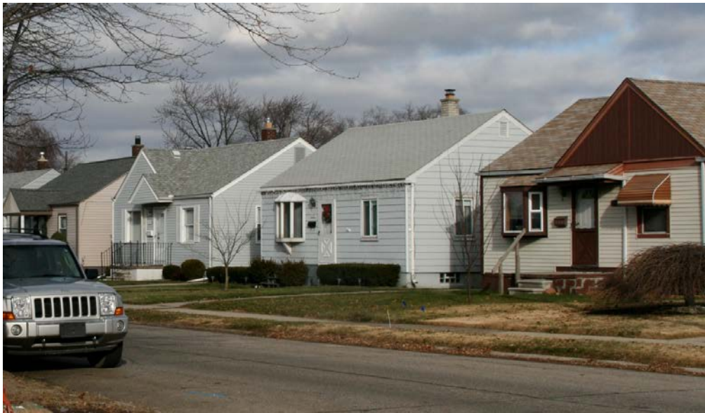
Figure 1. Typical existing houses in the NSP2 neighborhood
