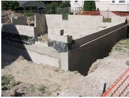
NSP2 Bid Pack 2 – New Construction 2011-06-28 – foundation complete
