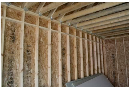
Garage framing at 16" on centre.
