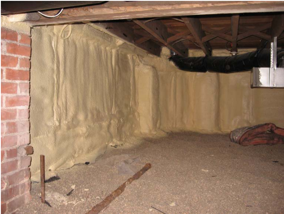
Figure 13. Spray foam installation in conditioned crawlspace at Cedar 1
