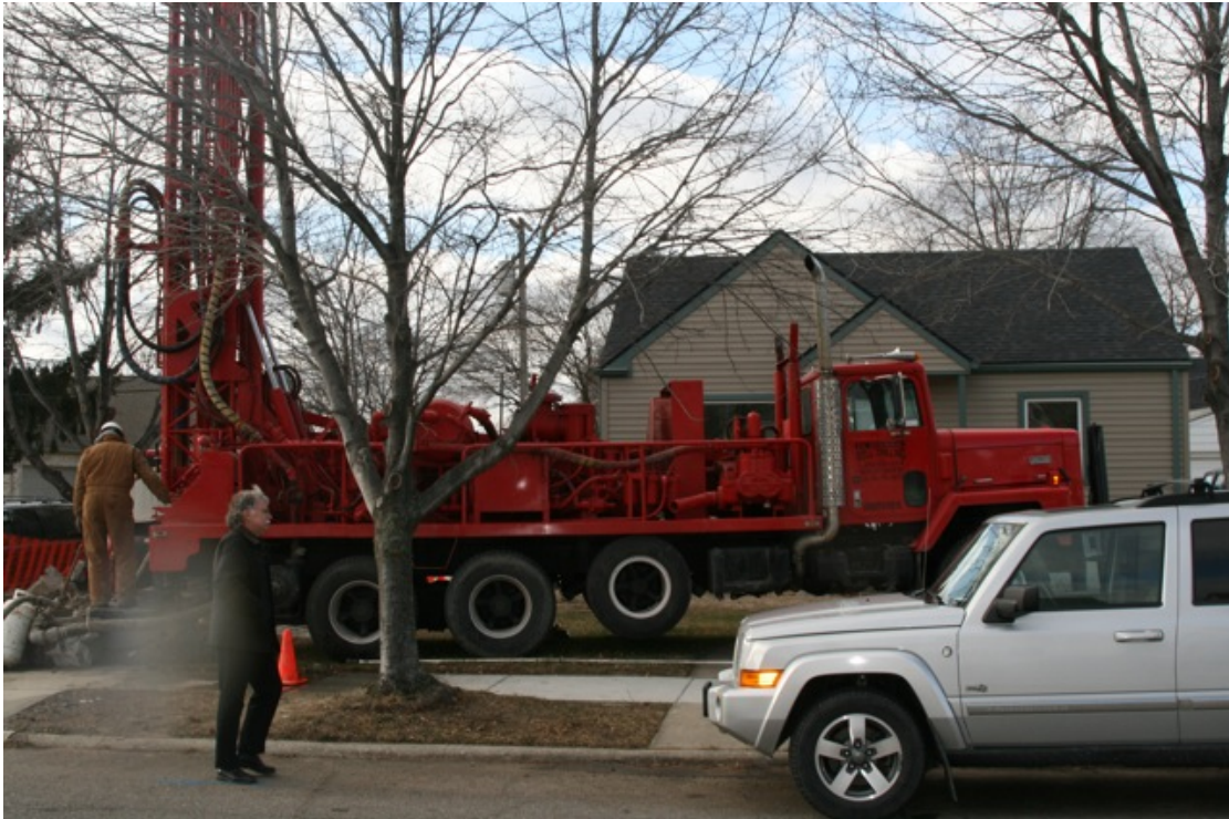
Figure 6. Photograph of a well operation for a GSHP system in the NSP2 neighborhood
