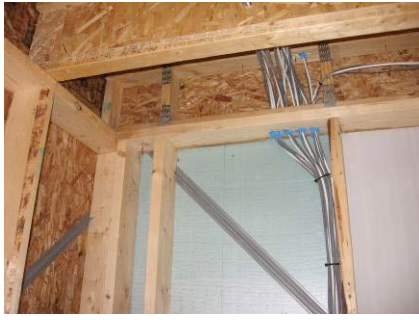
2011-10-06 – Mechanical and electrical work continues
