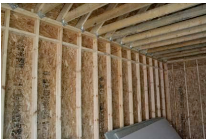
Garage framing at 16" on centre.
