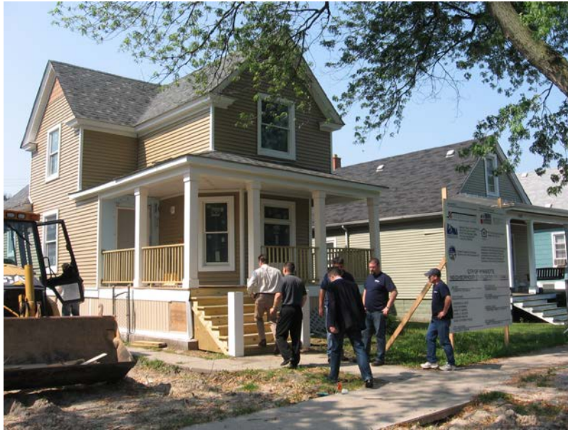
Figure 4. Photograph of Cedar 1 near completion
