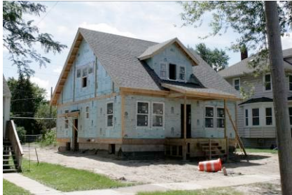
2011-08-22 – Framing nearing completion. Electrical, mechanical, and plumbing started
