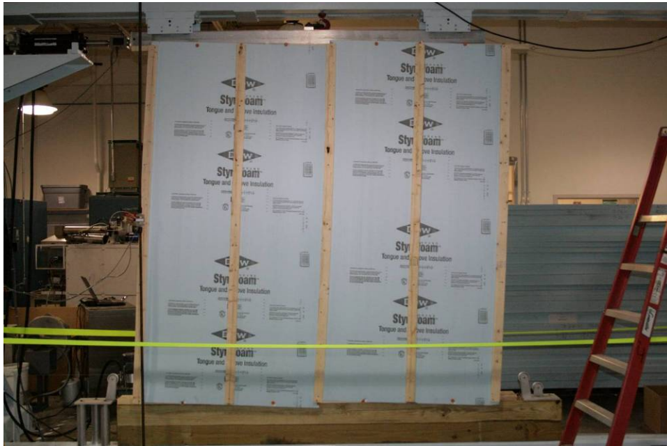
Figure 24. XPS sheets twisted in-plane
