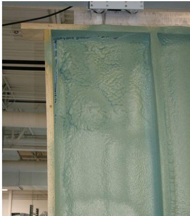
Figure 27. Stud flexure and ccSPF tearing
